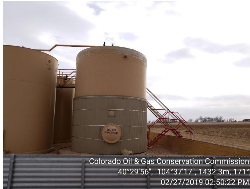
Photo 3: Produced Water tank with no placard
