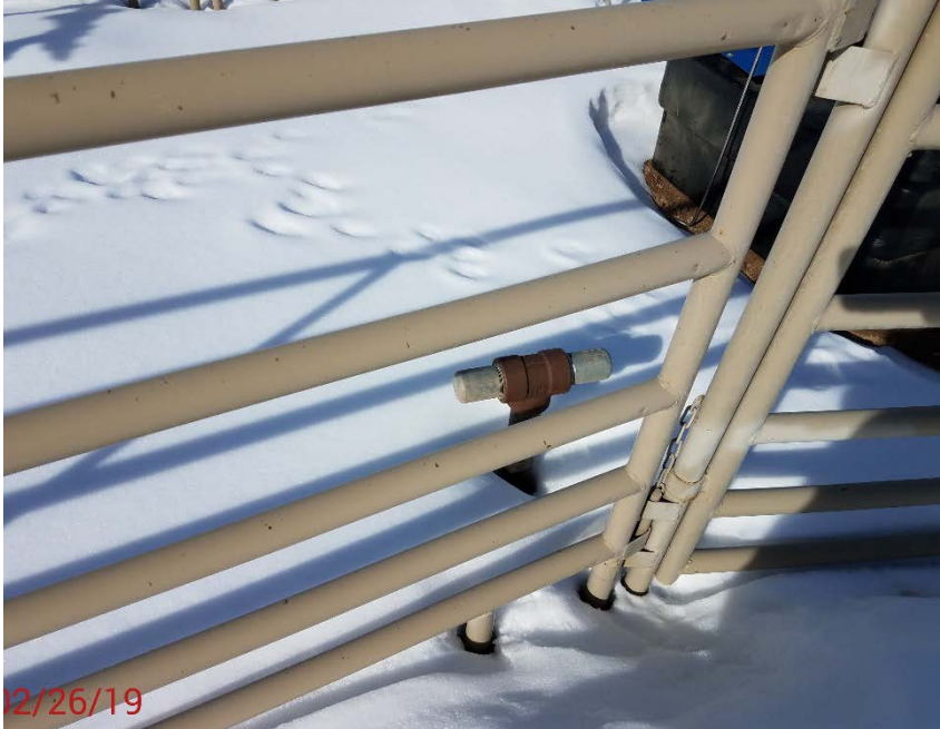
Location Photo #5, unused/unmarked flow line riser.
