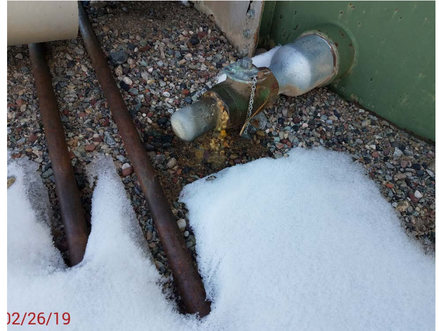
Location Photo #8, stained ground. Mechanical condition of 2" valve.
