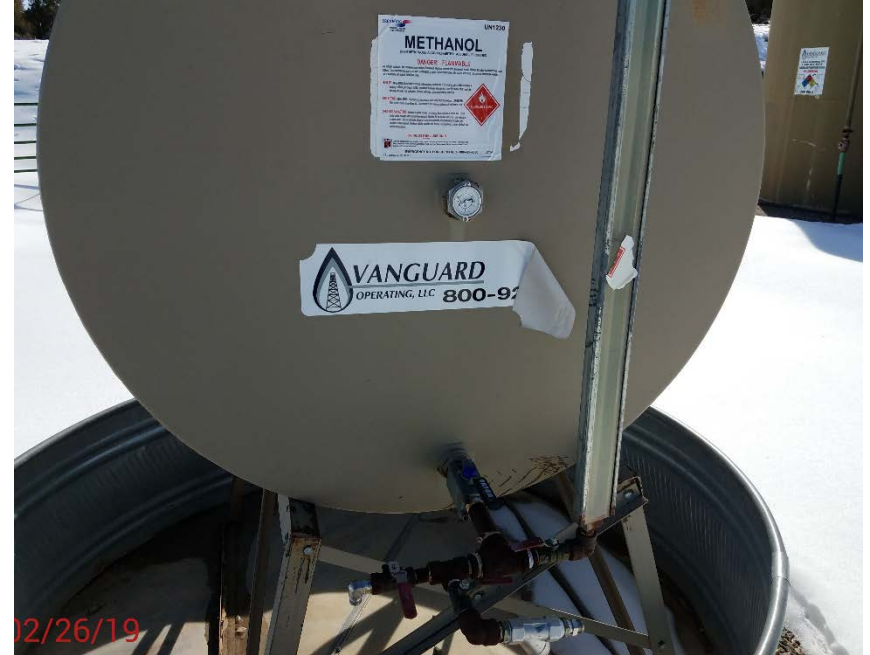
Location Photo #6, non legible sign on 500 gallon methanol tank.
