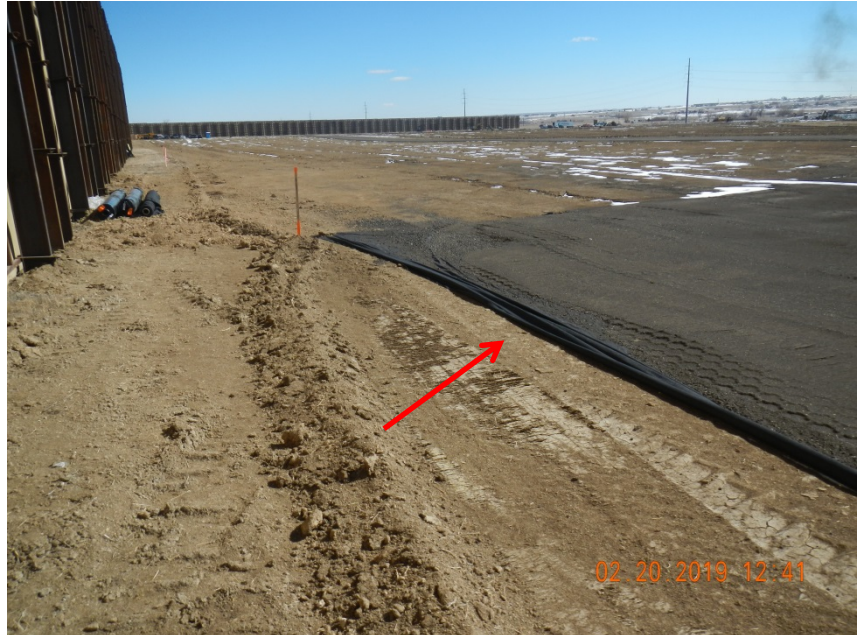
Photo 2. Photo taken from the northern perimeter of the location, facing East. Appears the operator has placed gravel over a geo textile fabric on top of the existing top soil.
