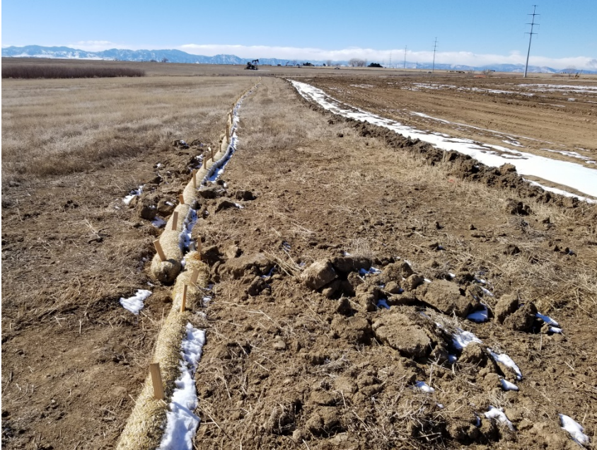
Photo 7. Photo taken from the southern perimeter of the location, facing West. Photo depicts BMP's installed around the parts of the southern perimeter of the location.
