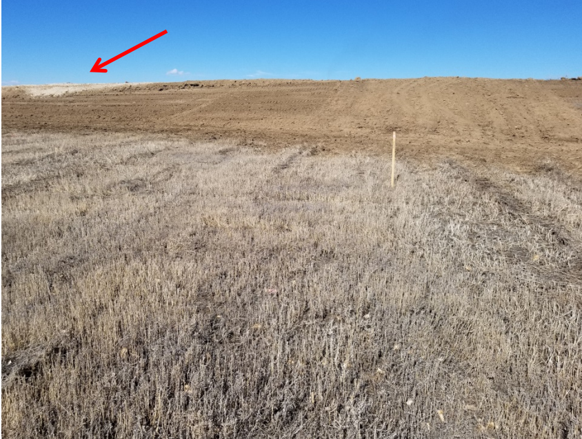
Photo 11. Photo taken from the southern perimeter of the location, facing North. Photo illustrates the second topsoil stockpile being stored along the southern area. Note the soil color change in the left of the photo. Appears the Operator was placing subsoil on top of the topsoil stockpile.
