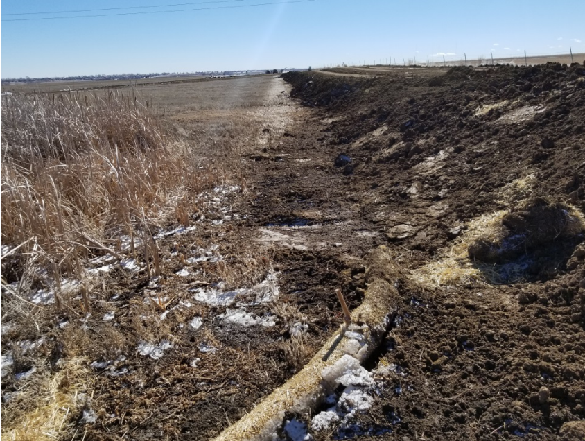
Photo 9. Photo taken from the western perimeter of the location, facing Southwest. Photo depicts BMP's have not been installed around the entire perimeter of the location and note the wetland on the left in the Photo.
