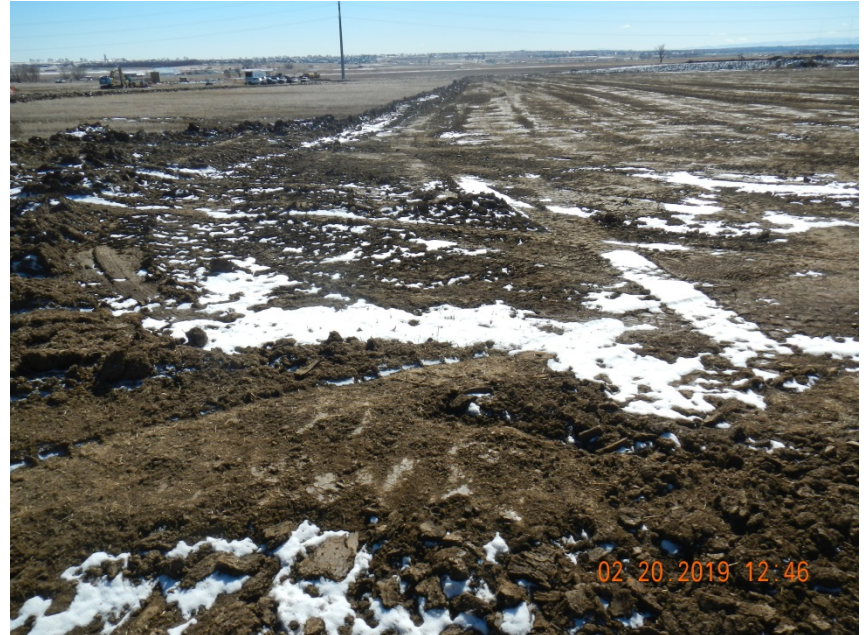
Photo 4. Photo taken from the northern perimeter of the location, facing South. Photo depicts potentially top soil not salvaged and that BMP's have not been installed around the entire perimeter of the location.
