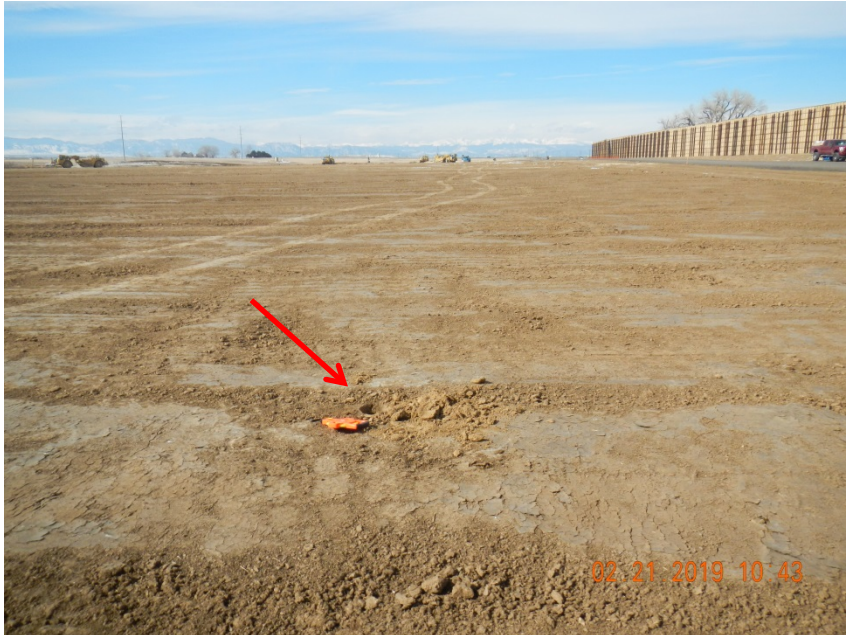
Photo 19. Photo taken from the eastern perimeter of the location, facing Southwest. Photo depicts 1 of 3 topsoil test pits taken on location in the disturbed area that topsoil salvage operations were said to be complete by the Operator.
