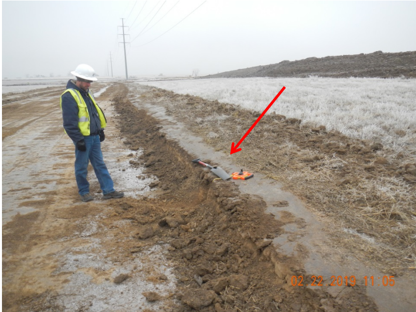
Photo 23. Photo taken from the southern perimeter of the location, facing West. Photo depicts a cut area where topsoil salvage operations were had been done by the Operator.
