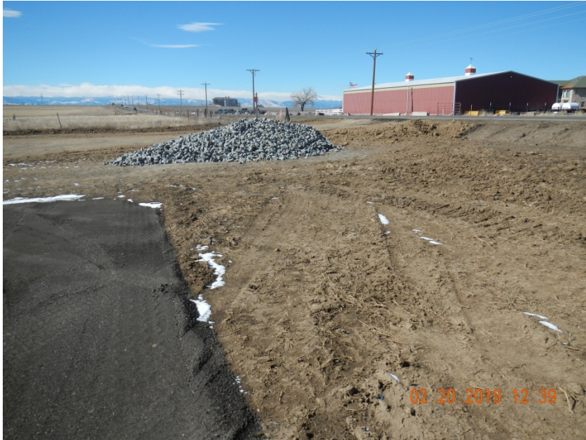
Photo 1. Photo taken from the northern perimeter of the location looking at the access road off CR 6, facing West. Operator is in the process of installing gravel to potentially to limit tracking onto the county road.
