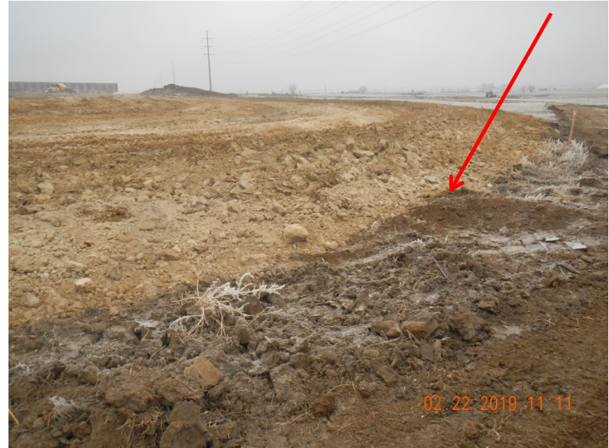
Photo 26. Photo taken from the southern perimeter of the location, facing North. Photo illustrates the area adjacent to the second topsoil stockpile being stored along the southern area. Note the soil color changes from the subsoil in the background to the topsoil in the foreground.
