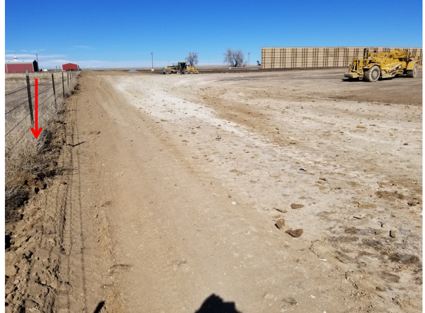
Photo 14. Photo taken from the western perimeter of the location, facing North. Photo depicts BMP's have not been installed around the entire perimeter of the location and note the wetland on the left in the Photo.
