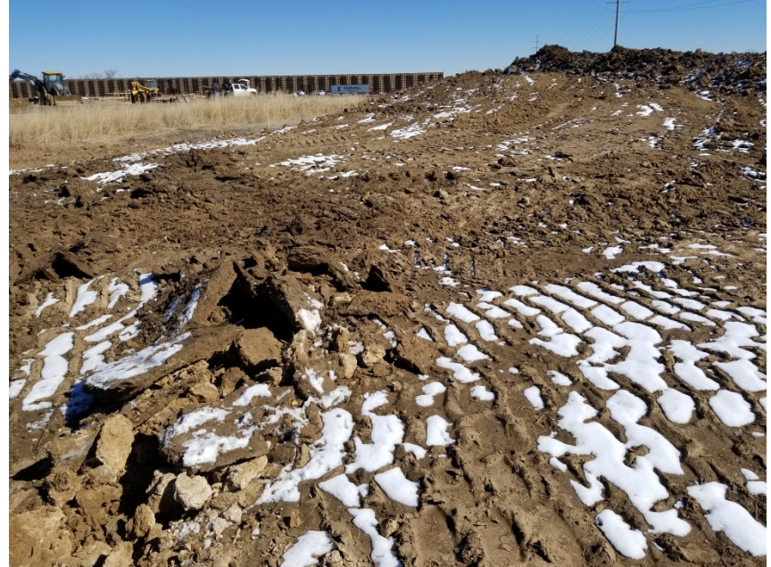
Photo 10. Photo taken from the Southern perimeter of the location, facing North. Photo illustrates a topsoil stockpile being stored along the southern area and is being temporarily stabilized with equipment tracking.
