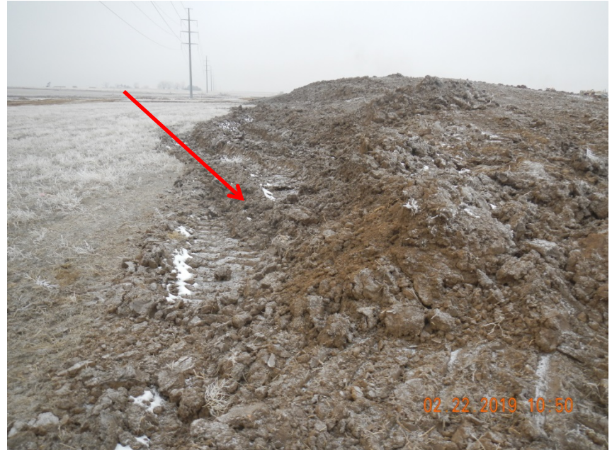
Photo 28. Photo taken from the southern perimeter of the location, facing West. Photo illustrates the first topsoil stockpile being stored along the southern area. Appears the Operator has not stabilized parts of the stockpile.
