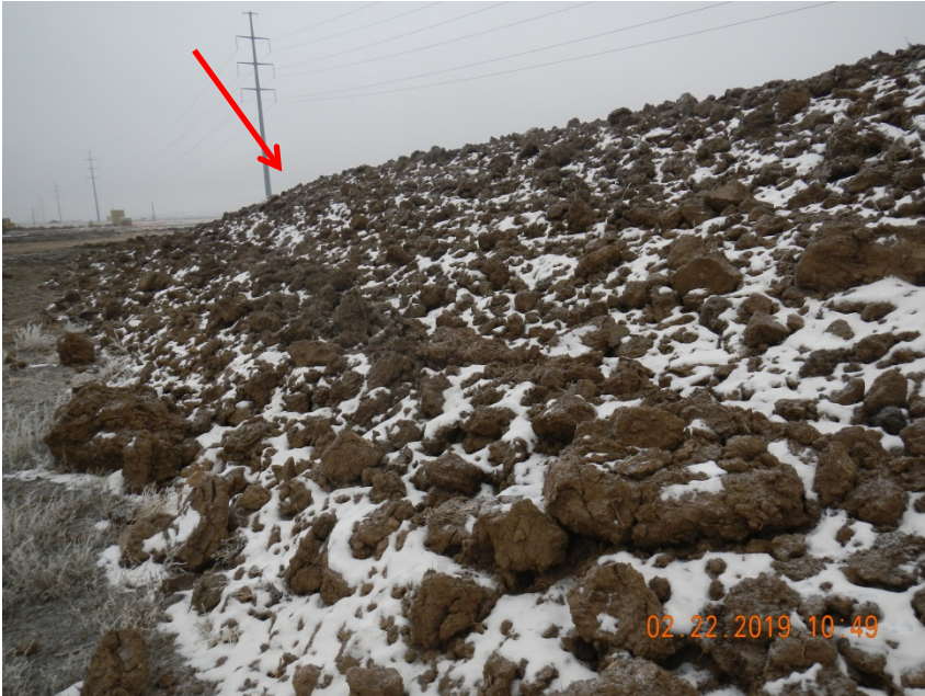
Photo 27. Photo taken from the southern perimeter of the location, facing East. Photo illustrates the first topsoil stockpile being stored along the southern area. Appears the Operator has not stabilized parts of the stockpile.
