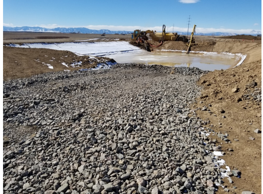
Photo 6. Photo taken from the Southern perimeter of the location, facing West. Photo depicts a temporary pond installed to fill water trucks.
