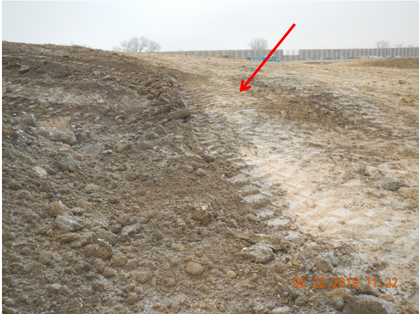
Photo 25. Photo taken from the southern perimeter of the location, facing North. Photo illustrates the second topsoil stockpile being stored along the southern area. Appears the Operator was still placing subsoil on top of the topsoil stockpile as of 2/22/2019.
