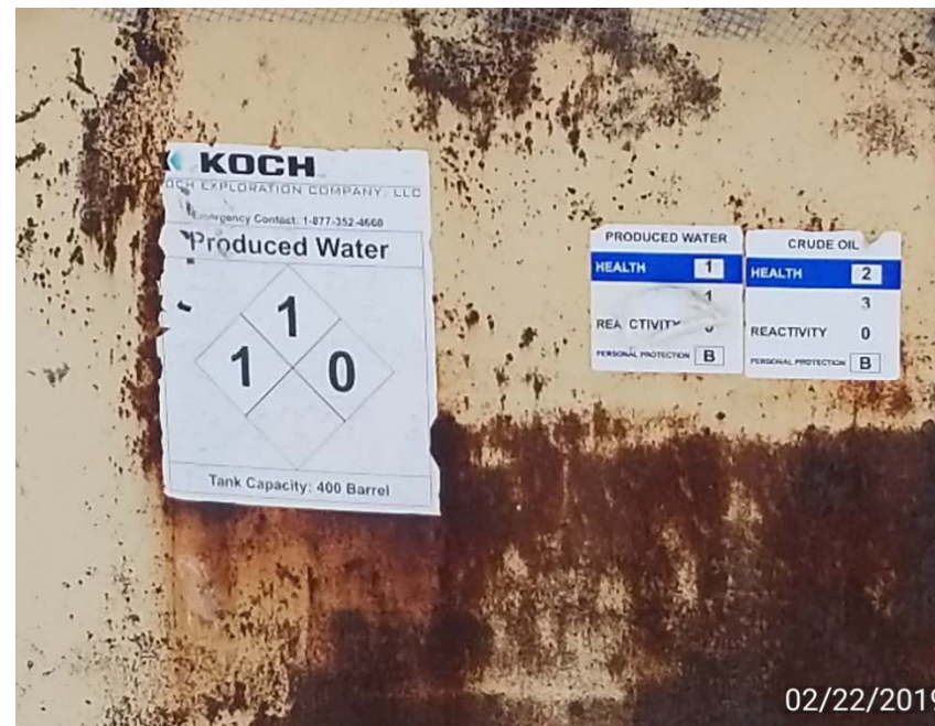
Photo 2. Blowdown tank does not have current operator and incorrect capacity.
