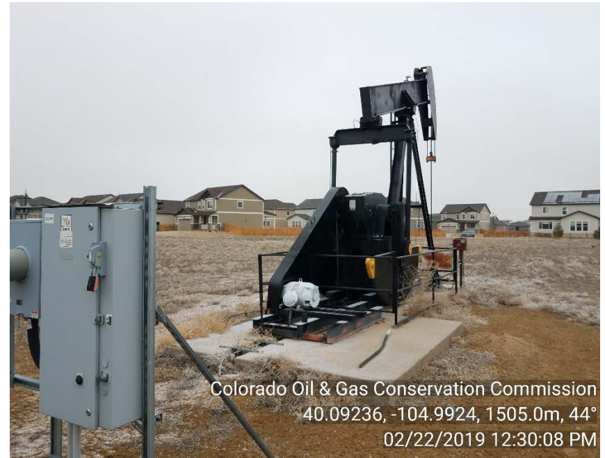
Electric disconnect and pump jack fencing
