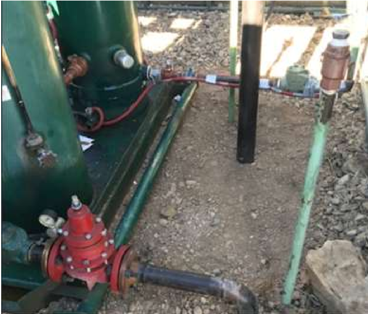
PHOTO 1: THE ACCUMULATED FLUID WAS REMOVED FROM THE LIQUID RING SKID.
