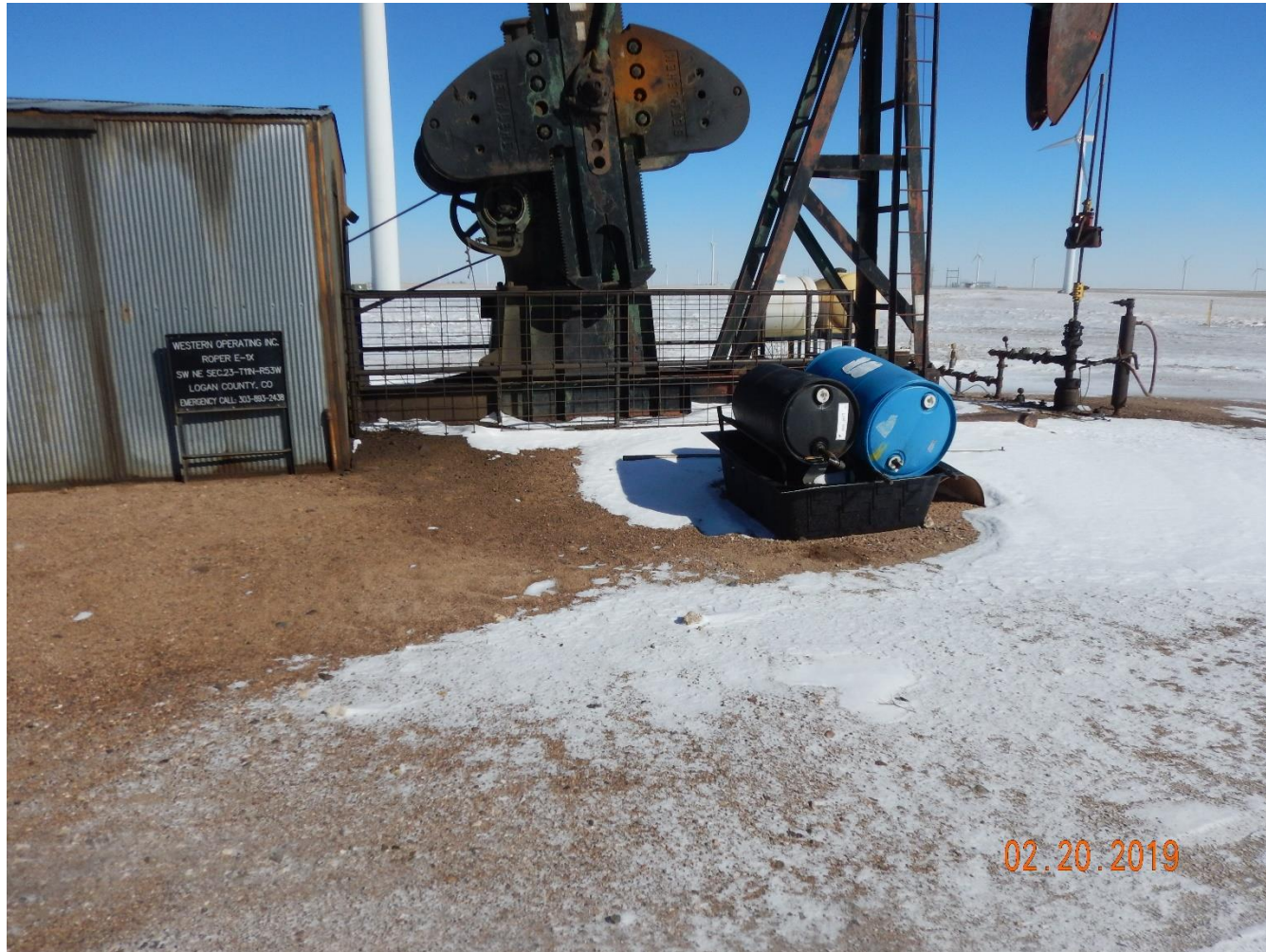
Photo 1: Photo taken from the south end of the well. Photo shows barrels have been placed into secondary containment.
