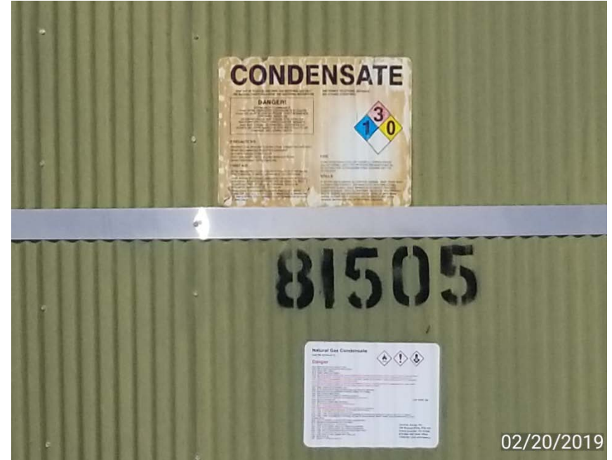
Photo 2. Tank sign missing capacity of 400 bbl.
