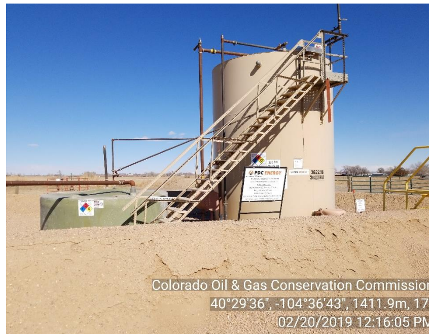
Photo 2: Tank Battery; no indication of capacity of Produced Water Tank.
