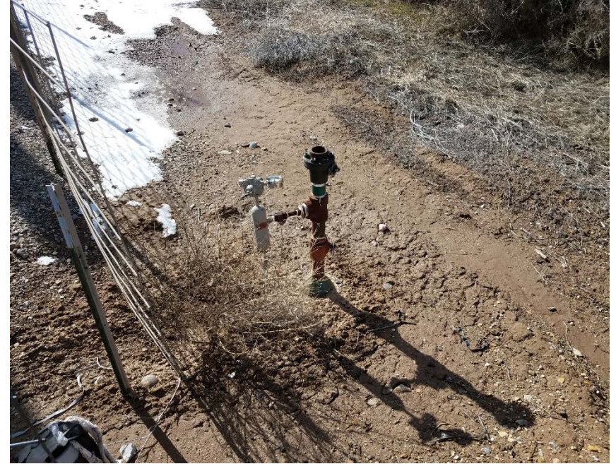
Location Photo #4, unmarked/unused flow line riser.
