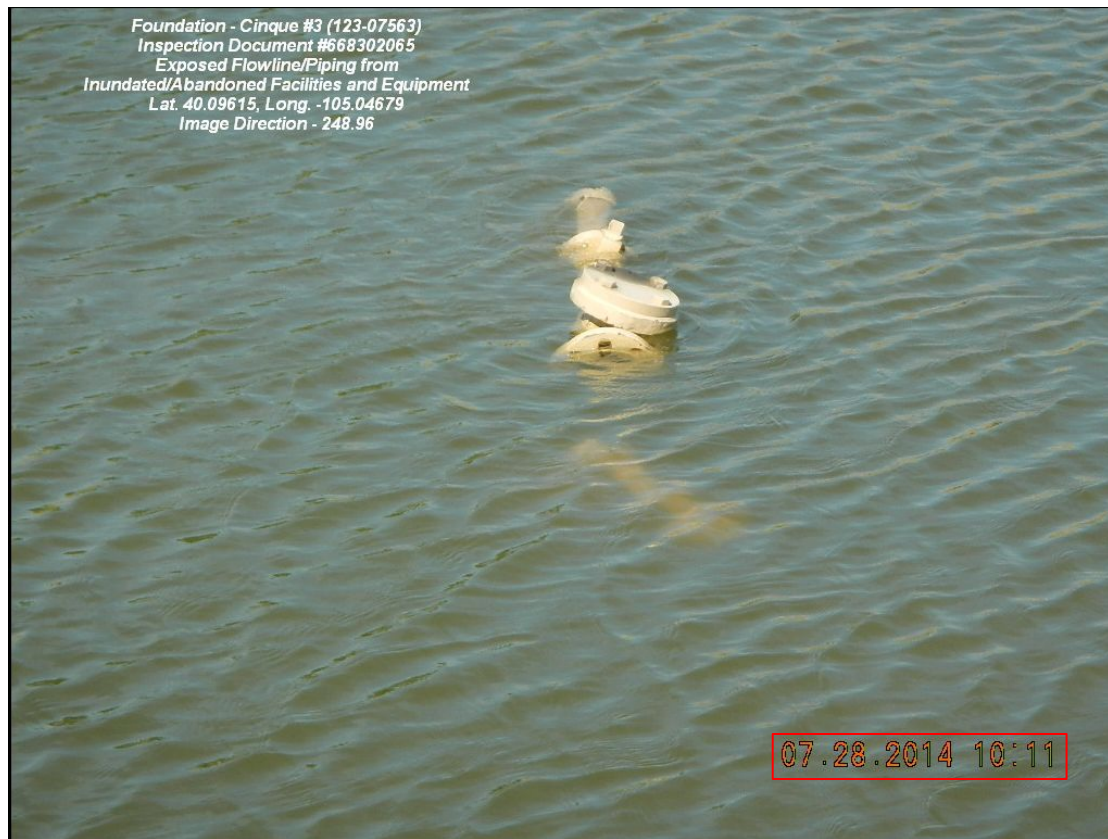
Photo 1. Photo taken 7/28/2014 from the abandoned facility illustrating unused equipment (exposed flowline/piping) submerged in water. A corrective action (CA) inspection was submitted to remove unused equipment, as well as other CA's.
