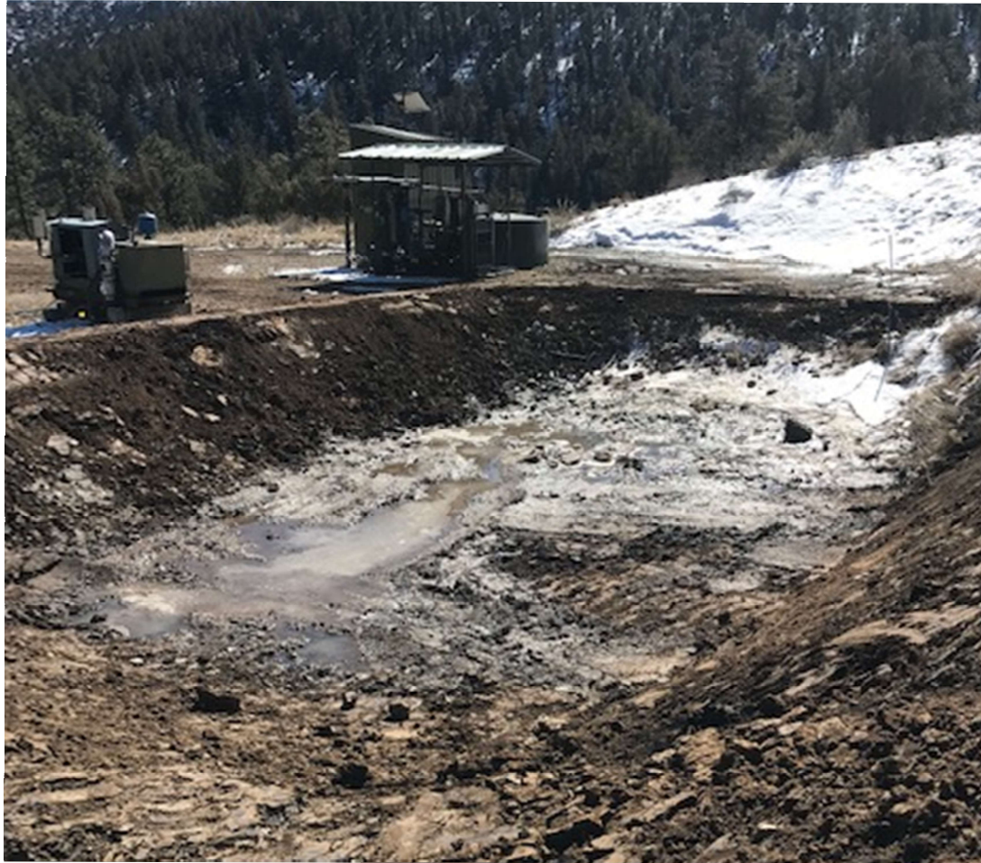
PHOTO 4: THE SOIL THAT SLOUGHED OFF INTO THE PIT WAS REMOVED.
