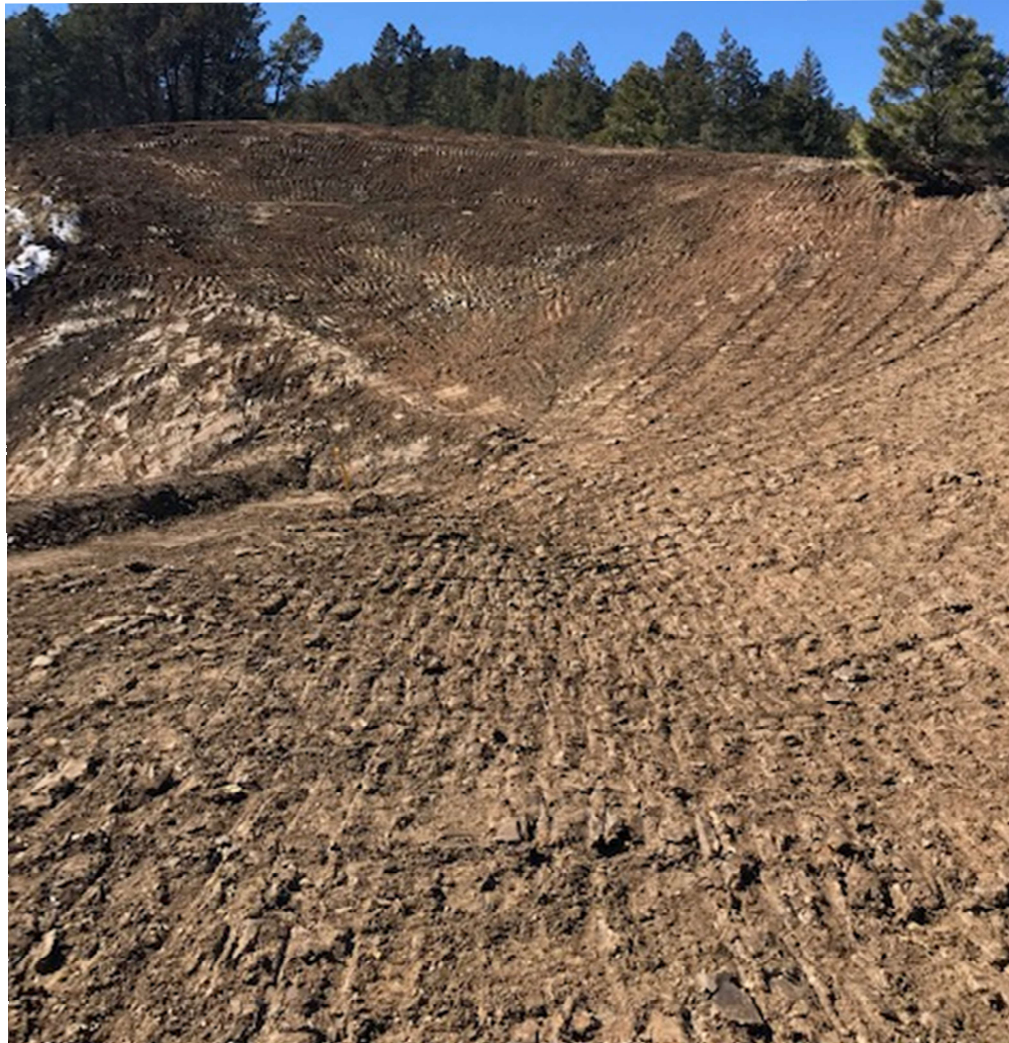
PHOTO 2: THE MATERIAL FROM THE PORTION OF THE CUT SLOPE THAT SLOUGHED OFF WAS REGRADED BACK TO THE ORIGINAL GRADE. GRADING TECHNIQUES WERE INSTALLED ON THE CONTOUR FOR TEMPORARY SOIL STABILIZATION. THE DISTURBED SOIL ON THE CUT SLOPE WILL BE HYDRO-SEEDED USING THE APPROVED COLORADO PARKS AND WILDLIFE SEED/SCRUB MIX, ALONG WITH FERTILIZER, SOIL ENHANCER & FLEXTERRA FLEXIBLE GROWTH MEDIUM DURING THE NEXT FAVORABLE GROWING SEASON.
