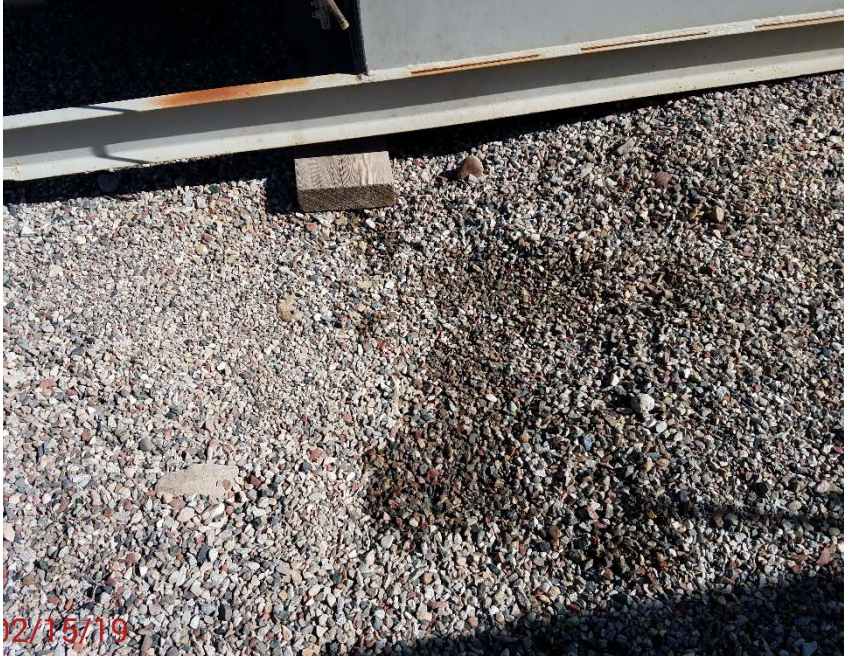
Location Photo #5, Stained material separator at blowdown line.
