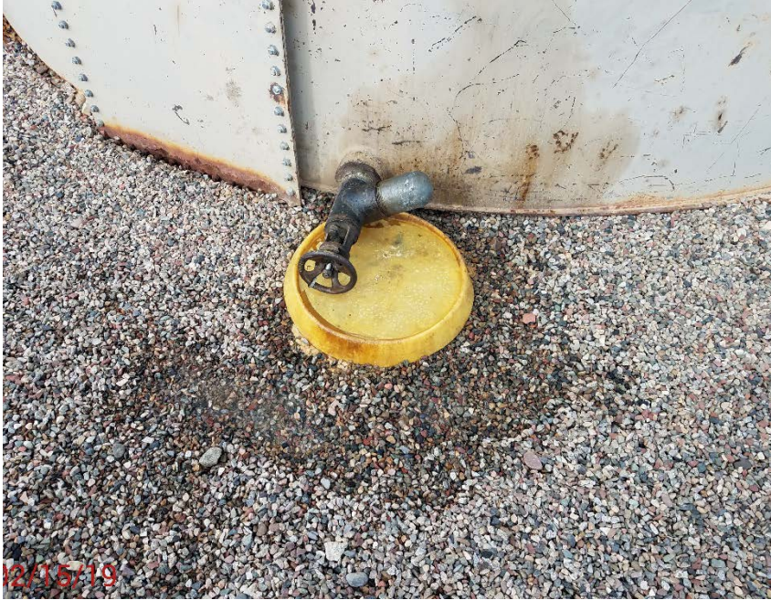
Location Photo #3, condensate in drip pan, stained material around drip pan.
