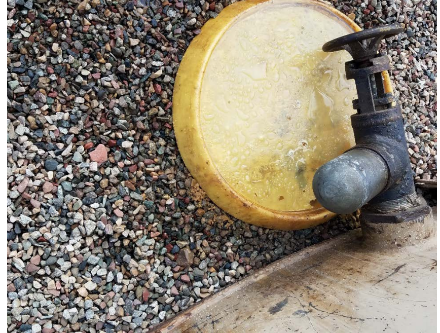
Location Photo #4, Stained material around drip pan.
