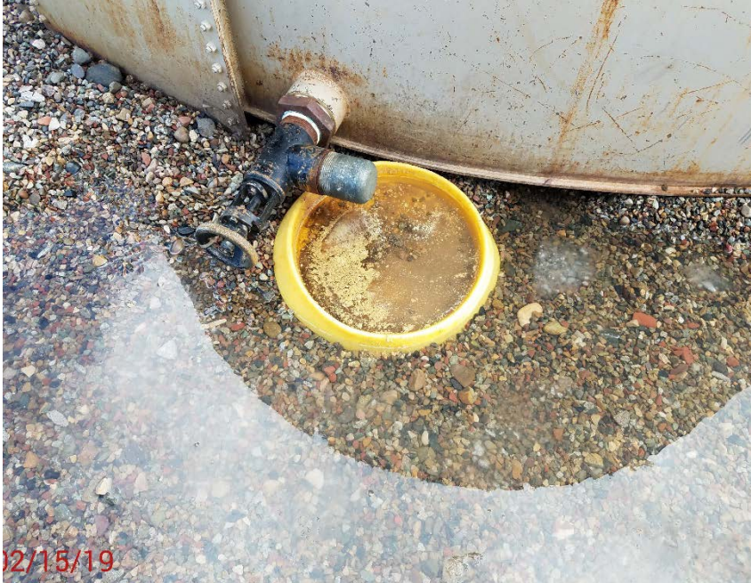
Location Photo #5, Condensate in drip pan.
