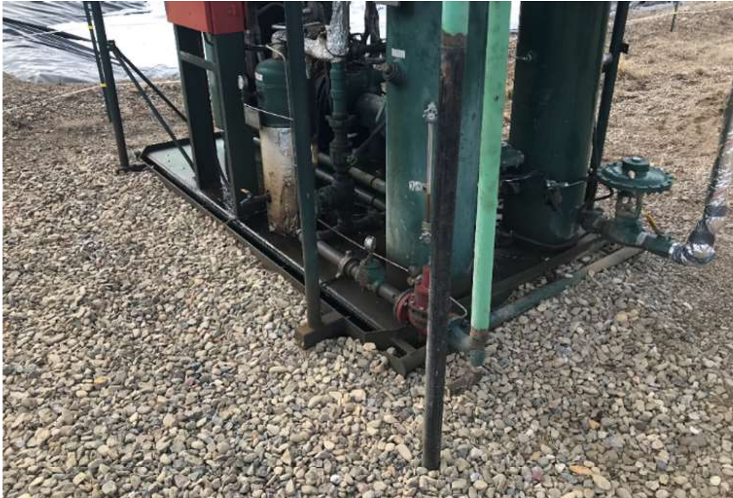
PHOTO 1: THE LIQUID RING SKID WAS CLEANED, THE FLUID ACCUMULATION WAS REMOVED FROM THE RESERVOIRS AND THE GROUND WAS CLEANED UP.
