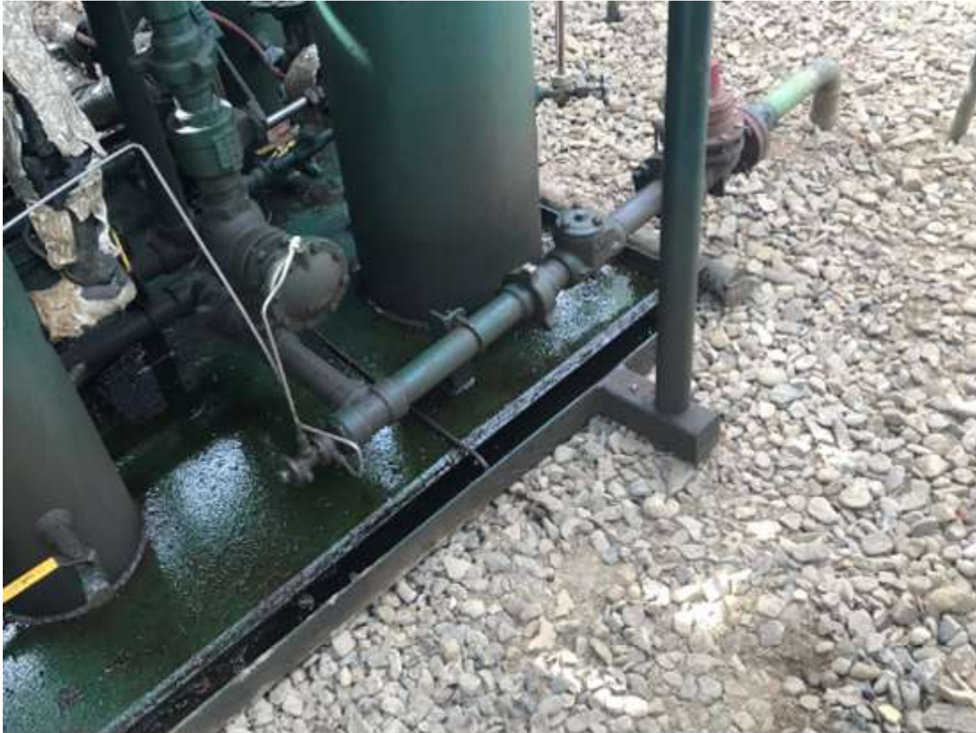
PHOTO 3: THE LIQUID RING SKID HAS BEEN CLEANED AND THE ACCUMULATED FLUID WAS REMOVED FROM THE RESERVOIR. THE STAINS ON THE GROUND HAVE BEEN CLEANED UP AS WELL.
