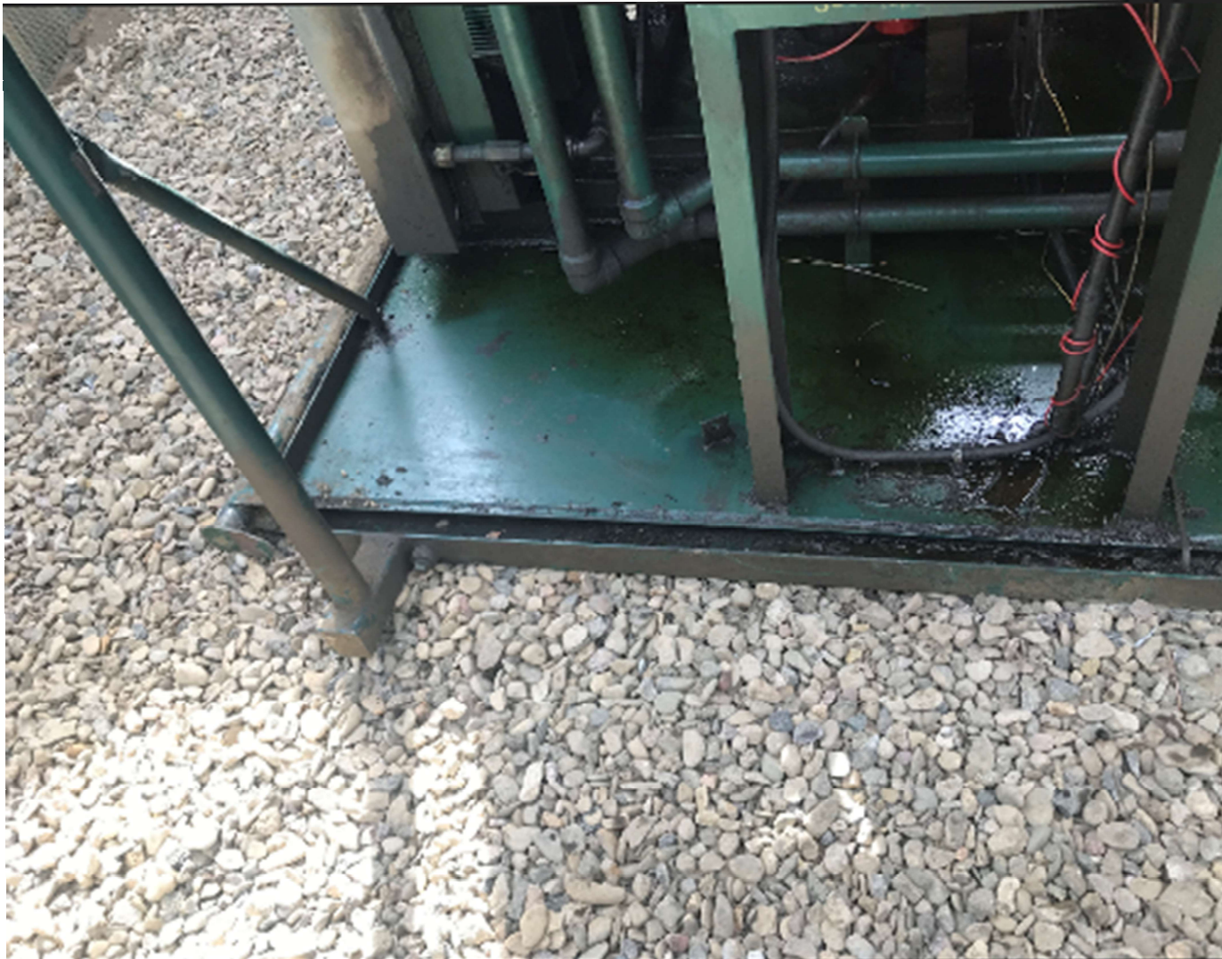
PHOTO 4: THE LIQUID RING SKID HAS BEEN CLEANED AND THE ACCUMULATED FLUID WAS REMOVED FROM THE RESERVOIR. THE STAINS ON THE GROUND HAVE BEEN CLEANED UP AS WELL.
