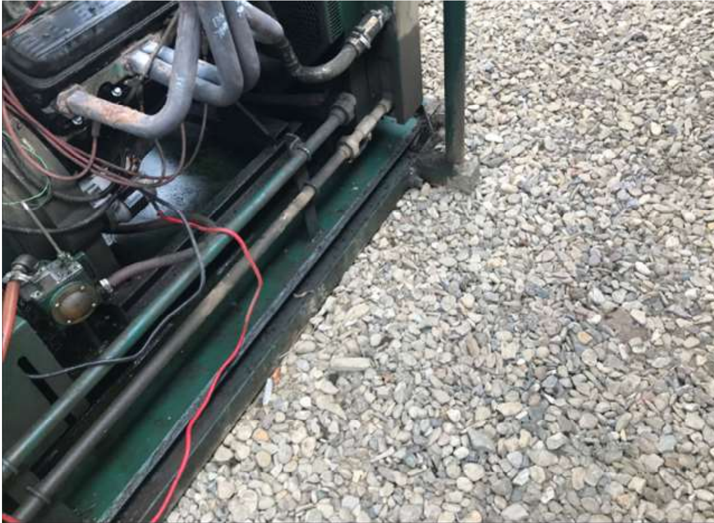
PHOTO 2: THE LIQUID RING SKID HAS BEEN CLEANED AND THE ACCUMULATED FLUID WAS REMOVED FROM THE RESERVOIR. THE STAINS ON THE GROUND HAVE BEEN CLEANED UP AS WELL.
