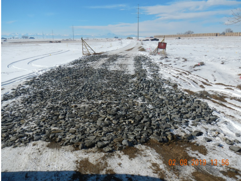
Photo 1. Photo taken from the access road looking into the location off CR 15, facing Northwest. Operator has installed gravel potentially to limit tracking onto the county road.
