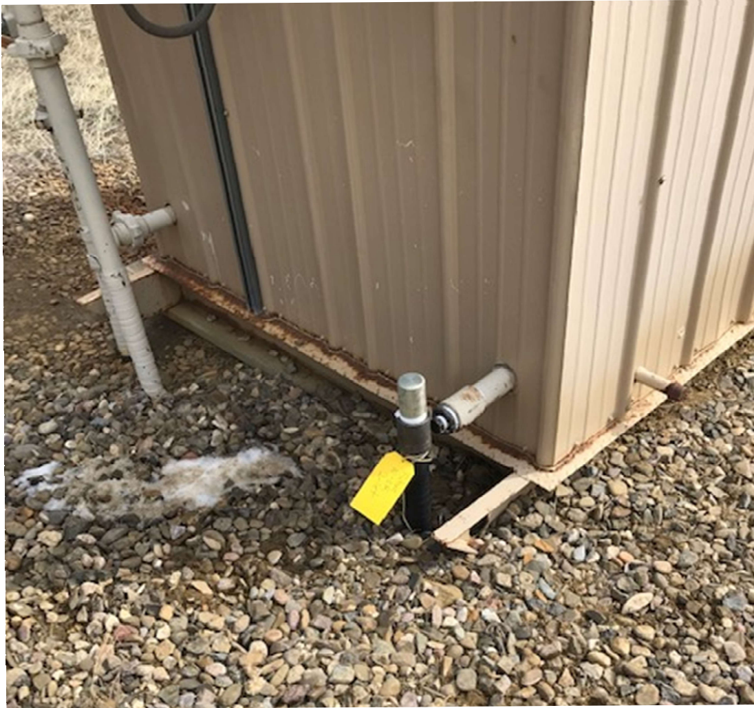
PHOTO 2: THE RISER WAS LABELED AND CAPPED.
