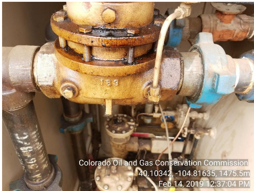
Photo 11 fluid on 2" piping inside sep house
