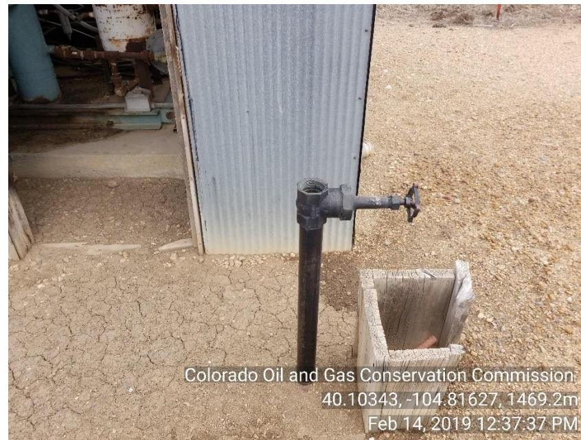
Photo 12 unused unmarked and not LOTO riser
