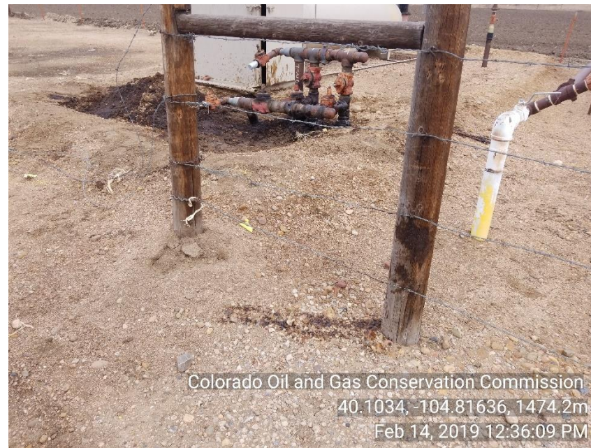
Photo 8 Stained soil in front of separator
