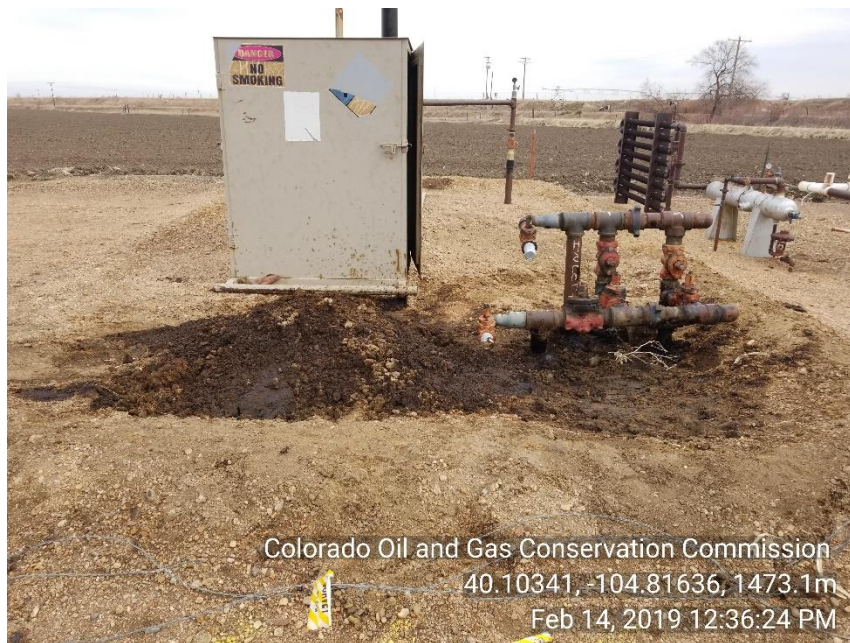
Photo 9 stained soil appeared to have leak in front of sep
