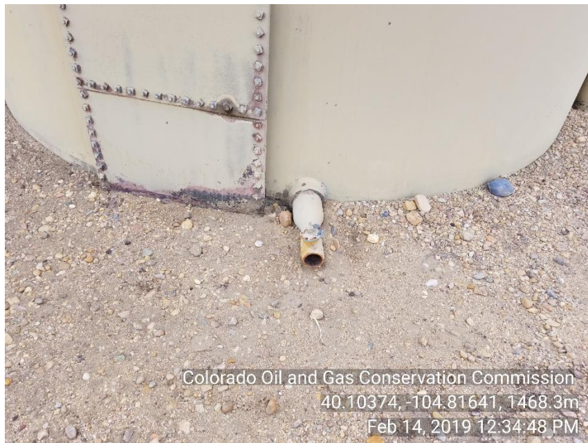
Photo 5 no bull plug crude oil tank load line
