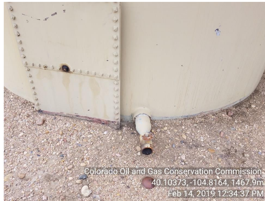
Photo 4 no bull plug on crude oil load line
