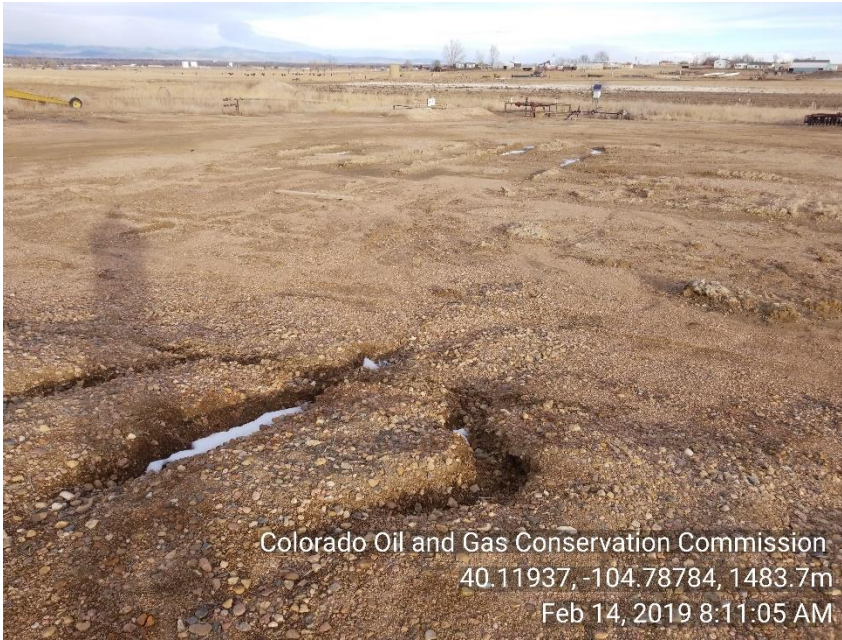
Photo 9 location does not have proper drainage reeling across location
