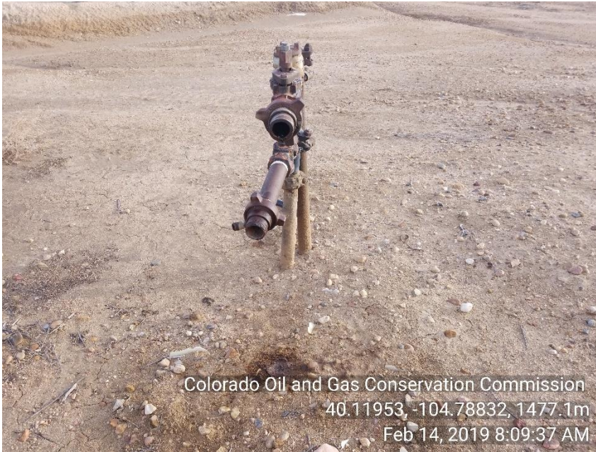
Photo 7 Unused, unmarked and not LOTO risers and stained soil
