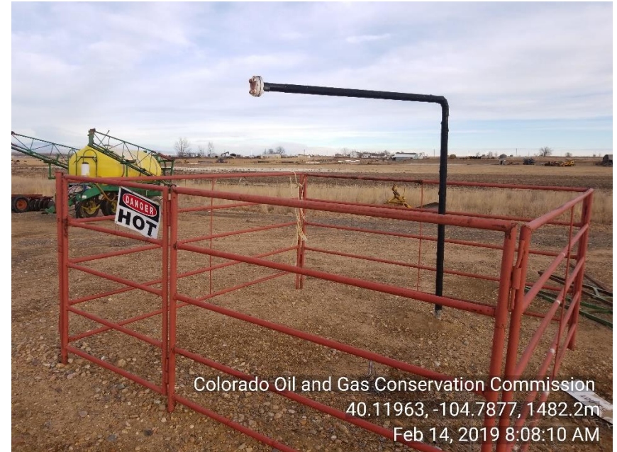
Photo 4 Unused unmarked and not LOTO riser
