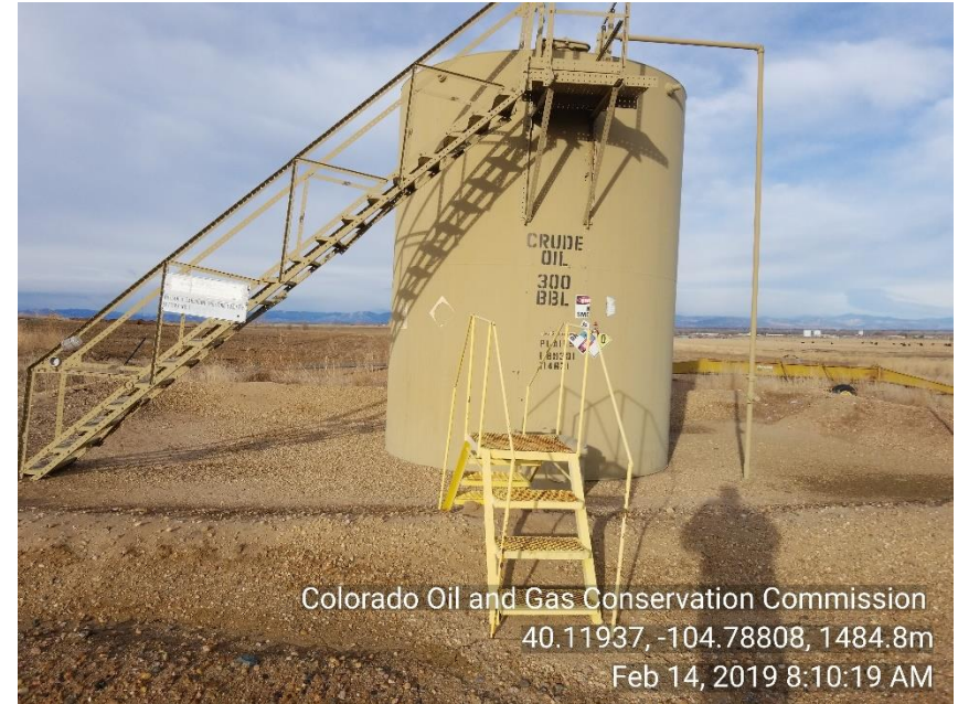
Photo 8 TNK BTRY Loc sign faded, NFPA placards torn off
