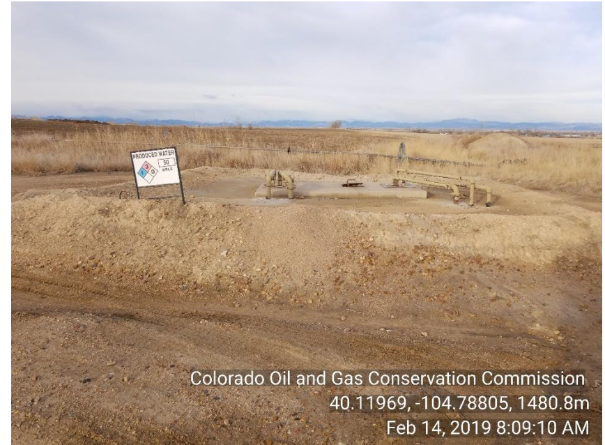
Photo 6 Produced water tank. Berms not adequate and in disrepair.
