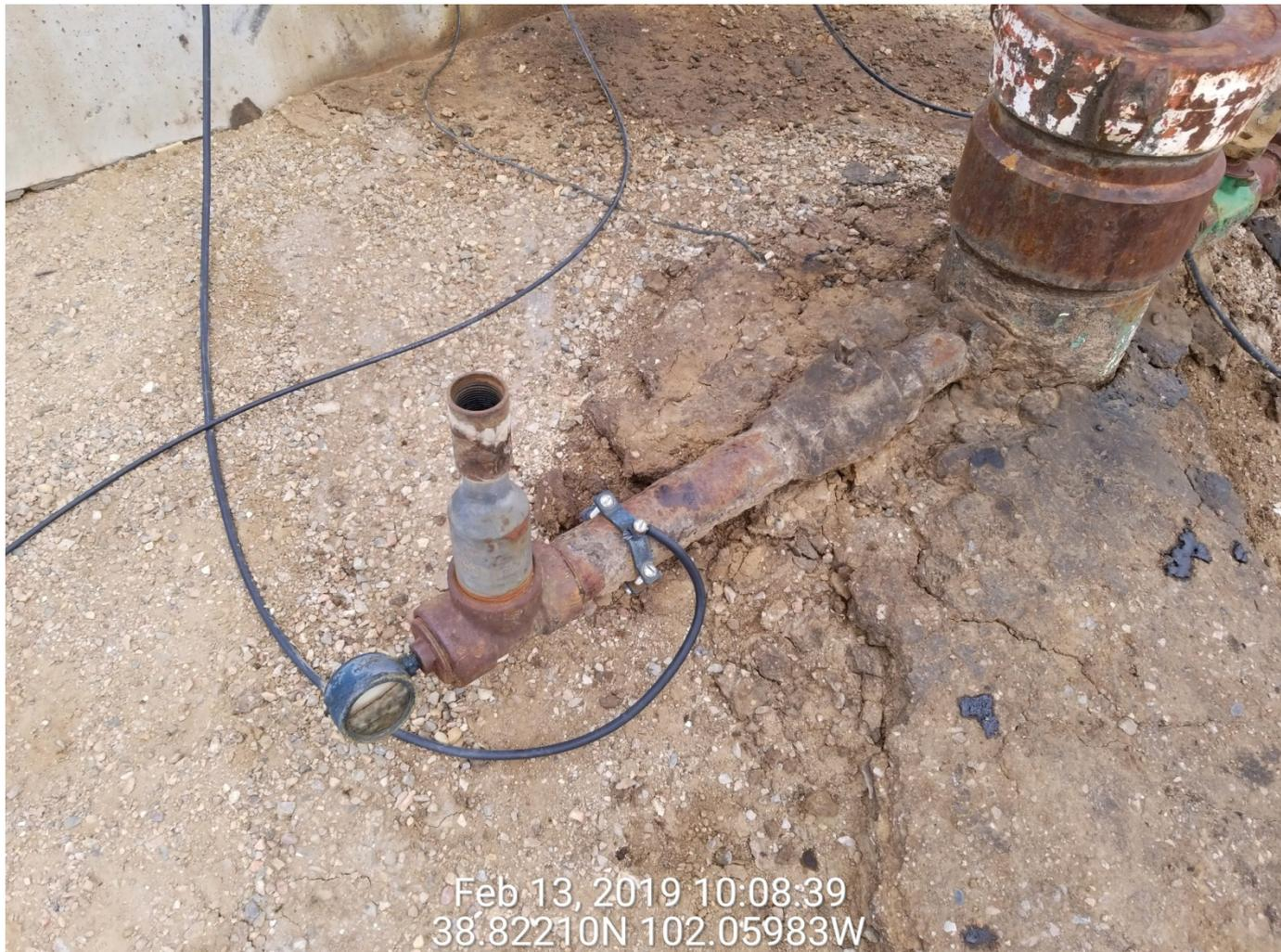
Valve that was observed to be venting during my last inspection has been removed leaving this open pipe that was observed to be actively venting methane gas.
