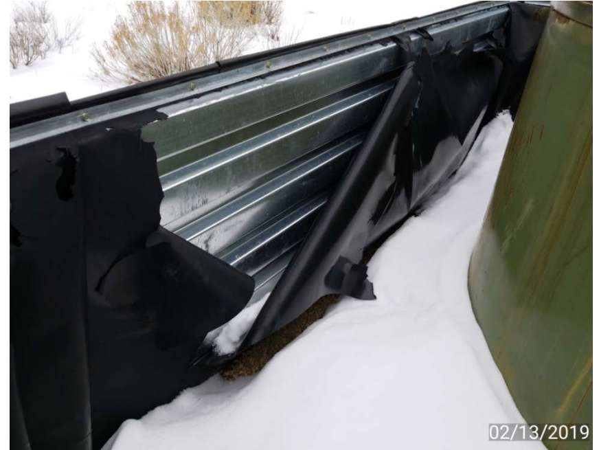
Photo 2. Liner failing on tank secondary containment.
