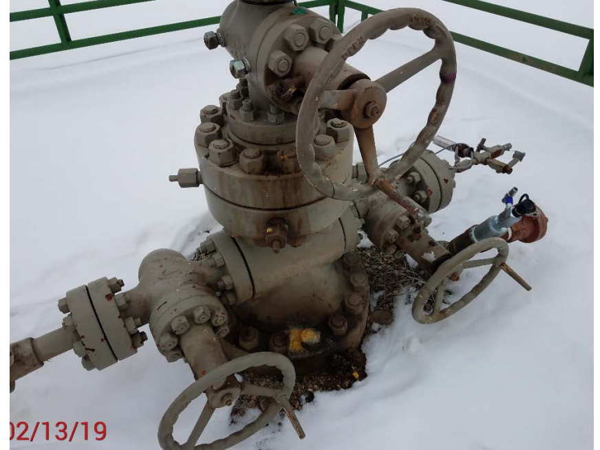
Location Photo #4, Mechanical condition of master valve.
