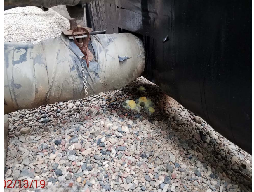
Location Photo #6, Stained ground under tank valves, mechanical condition of pipe fittings. Condensate on ground.
