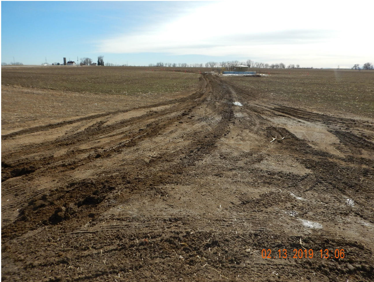
Photo 1. Photo taken from the entrance of the location off Niwot Rd., facing South. No tracking device BMP's installed or not adequately maintained to prevent track of material offsite.
