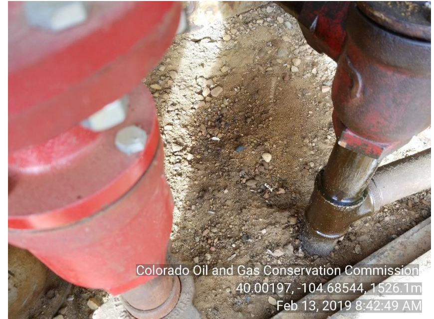
Photo 16 leaking fitting and stained soil inside separator
