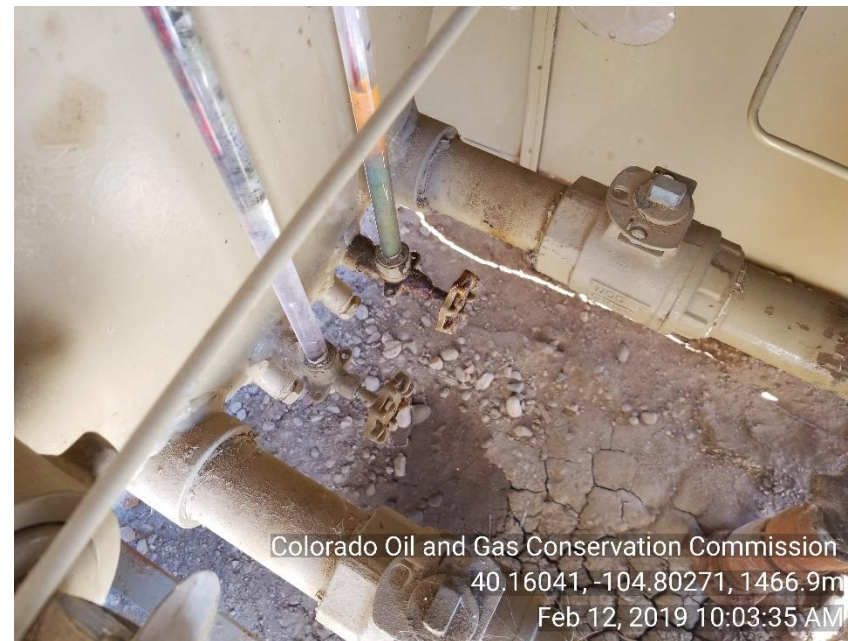
Photo 12 Leaking VLV on sight glass and stained soil inside SEP
