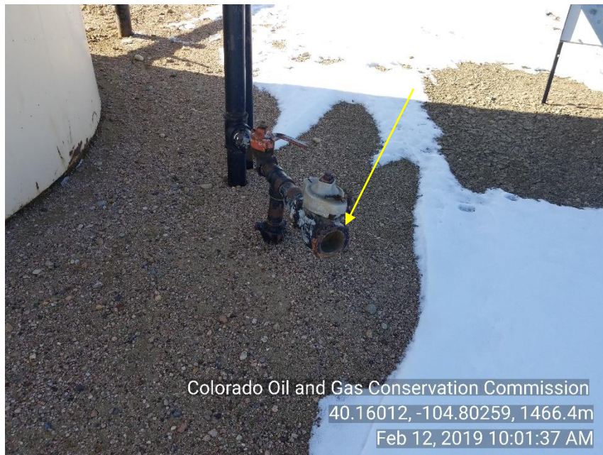
Photo 9 Load line to crude oil tank not bull plugged
