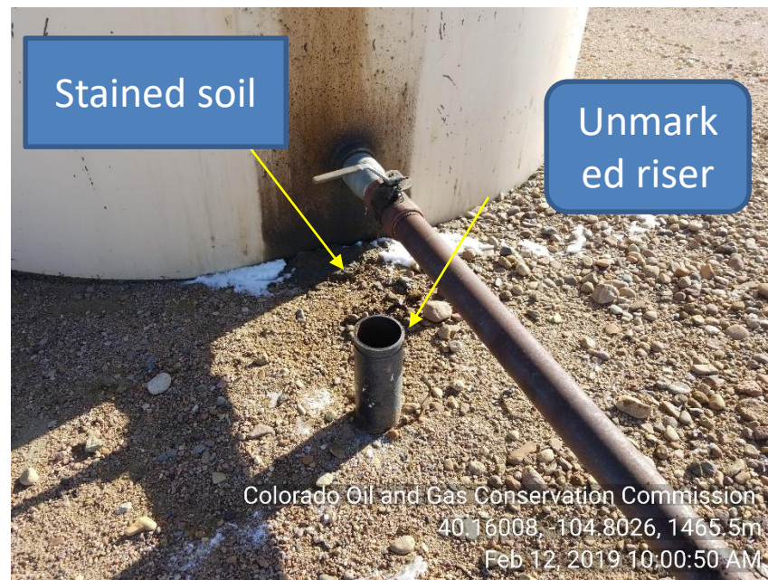
Photo 6 Stained soil. Unmarked riser not plugged or LOTO
