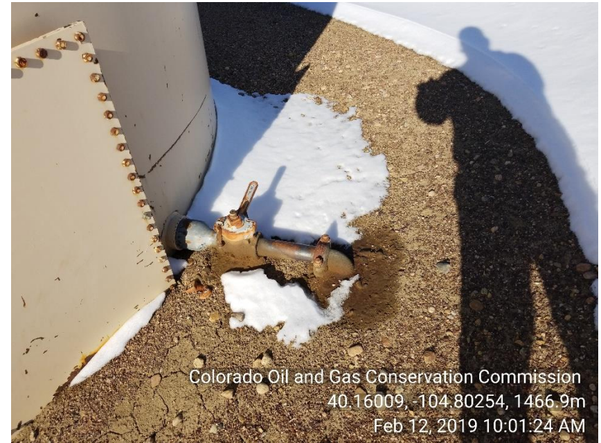
Photo 8 Stained soil in back of crude oil tank
