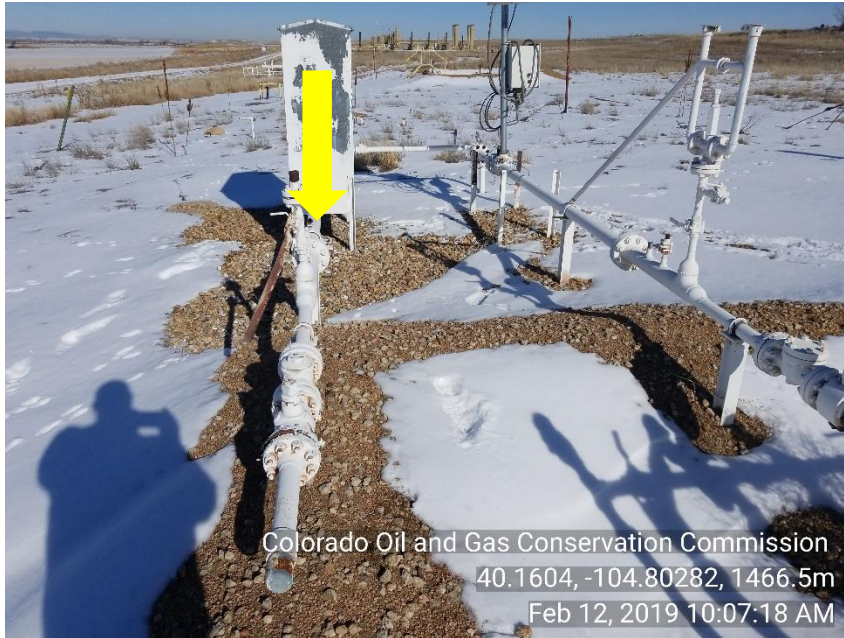
Photo 15 Unused equipment unused meter run
