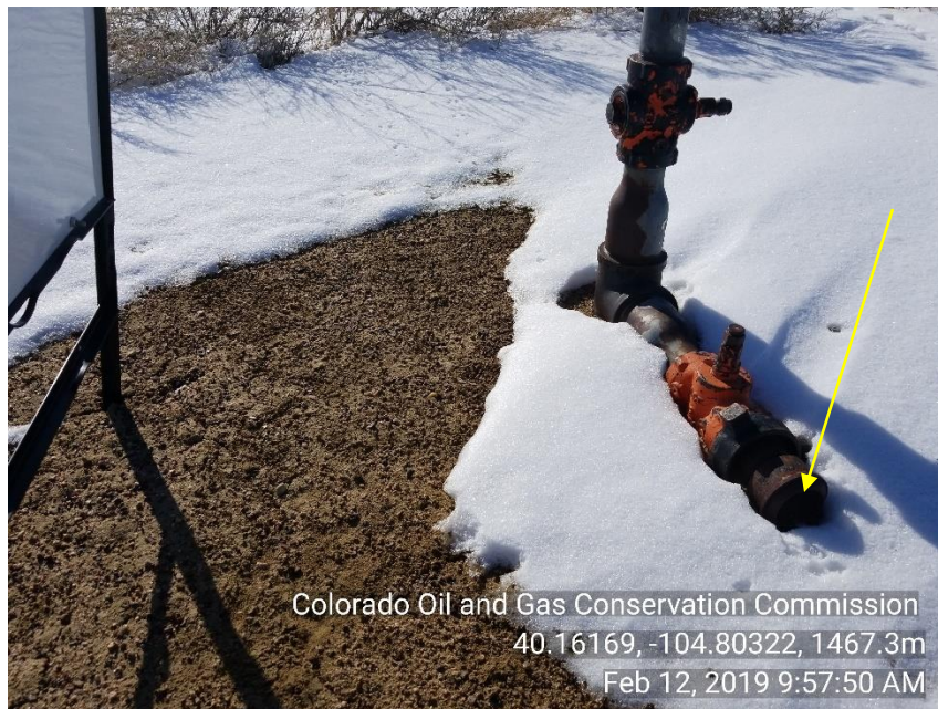
Photo 3 Unmarked riser not plugged or LOTO
