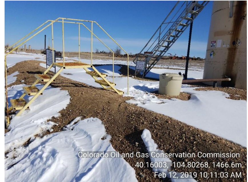
Photo 16 berms inadequate
