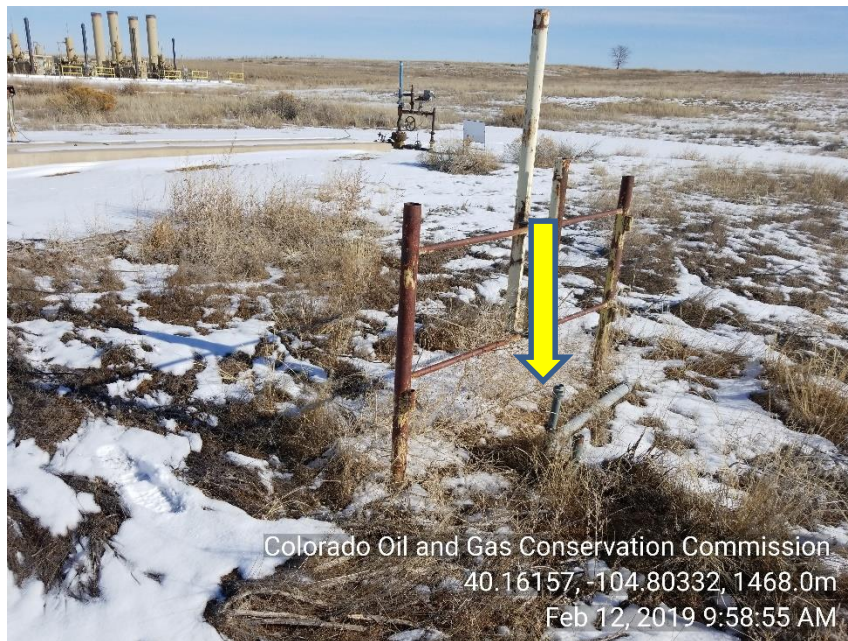
Photo 5 Unmarked riser not plugged or LOTO
