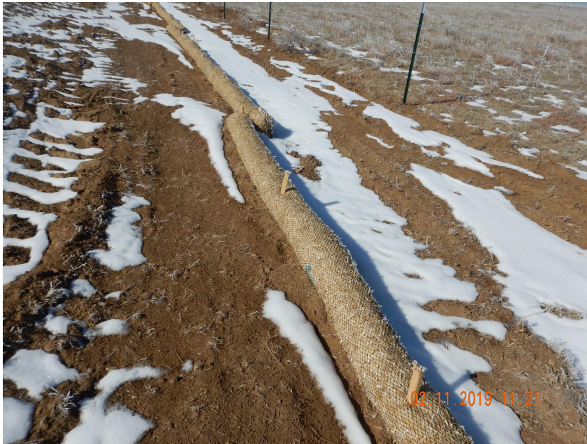
Photo 13. Close up photo taken from the northeastern perimeter of location, facing West. Straw wattles have not been properly installed (i.e., trenched).
