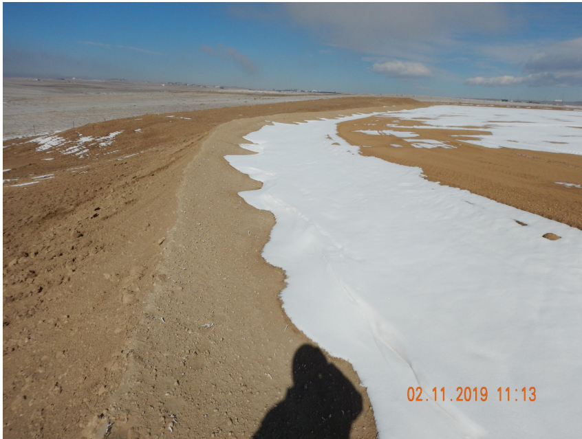
Photo 7. Photo taken from the southwestern well pad, facing North. Photo illustrates an unconsolidated berm that has been installed around the western, northern and eastern well perimeter. Operator shall properly stabilize berm BMP.
