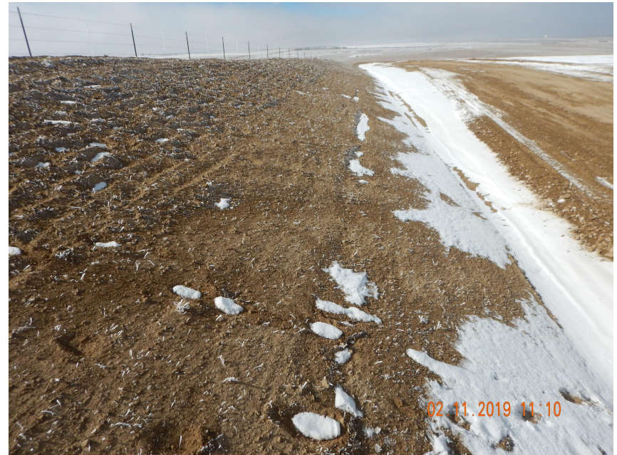
Photo 6. Photo taken from the southern cut slope, facing West. Operator shall properly stabilize all cut and fill slopes for long-term stabilization. Cut and fill slopes have been temporarily stabilized with equipment tracking.
