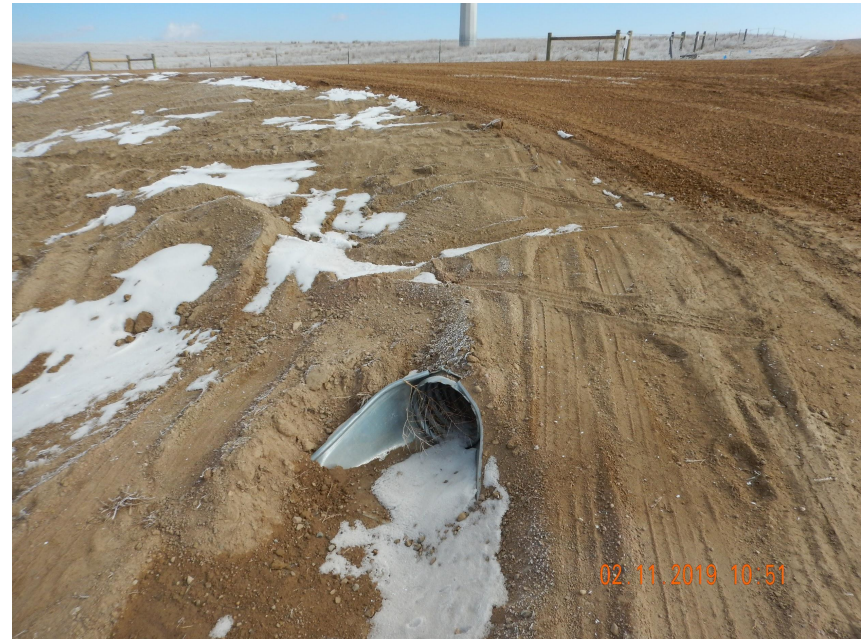
Photo 2. Photo taken from the entrance of location, facing East. Photo illustrates a culvert that has been installed in conjunction with the road side ditch.
