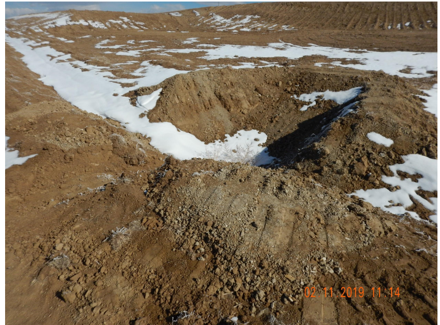
Photo 8. Photo taken from the southwestern perimeter of location, facing Northeast. Sediment trap is in-process of being constructed. If this is the only planned stabilized outlet for the location, this is not constructed to a sufficient size for an approximate 10 acre well pad.
