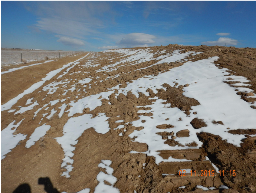
Photo 9. Photo taken from the southern topsoil stockpile, facing North. Photo illustrates the topsoil has been temporarily stabilized with equipment tracking. Operator shall stabilize the topsoil stockpile for long-term stabilization and to protect the topsoil from weed establishment.
