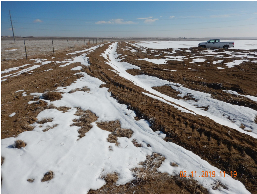
Photo 11. Photo taken from the northwestern perimeter of location, facing East. Photo illustrates a ditch and berm BMP that has been installed which is currently only directed to one stabilized outlet.
