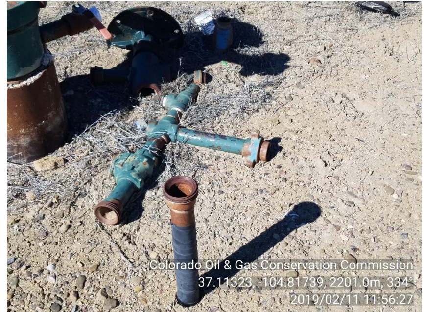
PHOTO 4: UNUSED UNMARKED RISER NOT LO/TO, UNUSED EQUIPMENT STORED ON LOCATION.
