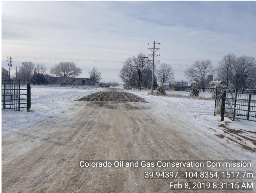
Photo 7 Tracking pad into location
