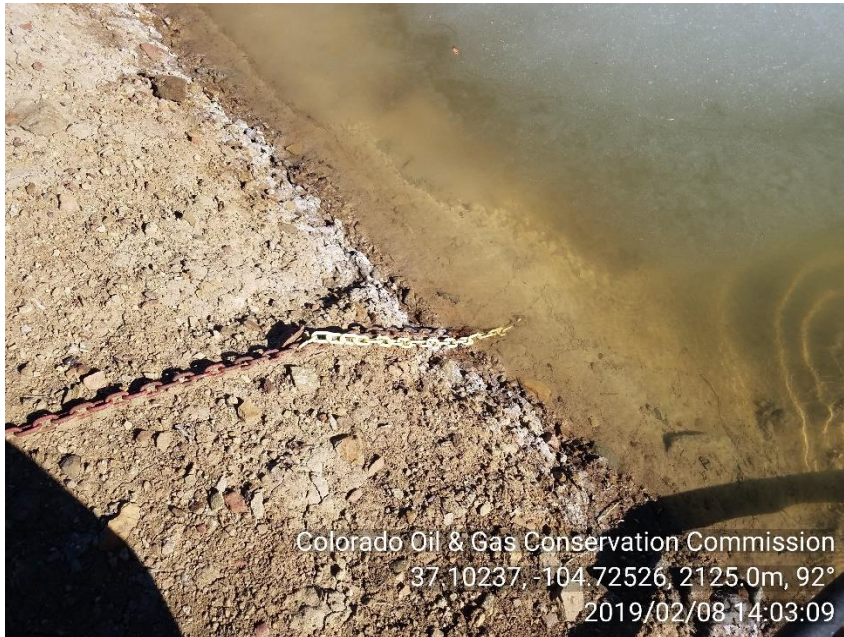
PHOTO 3: PRODUCED WATER LEVEL IN PIT IS ABOVE 2' FREEBOARD MARKER
