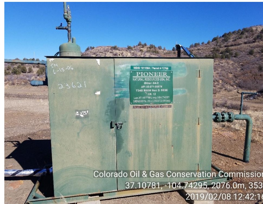
PHOTO 2: WELL SIGN/METER HOUSE/EMERGENCY CONTACT NUMBER NOT LEGIBLE
