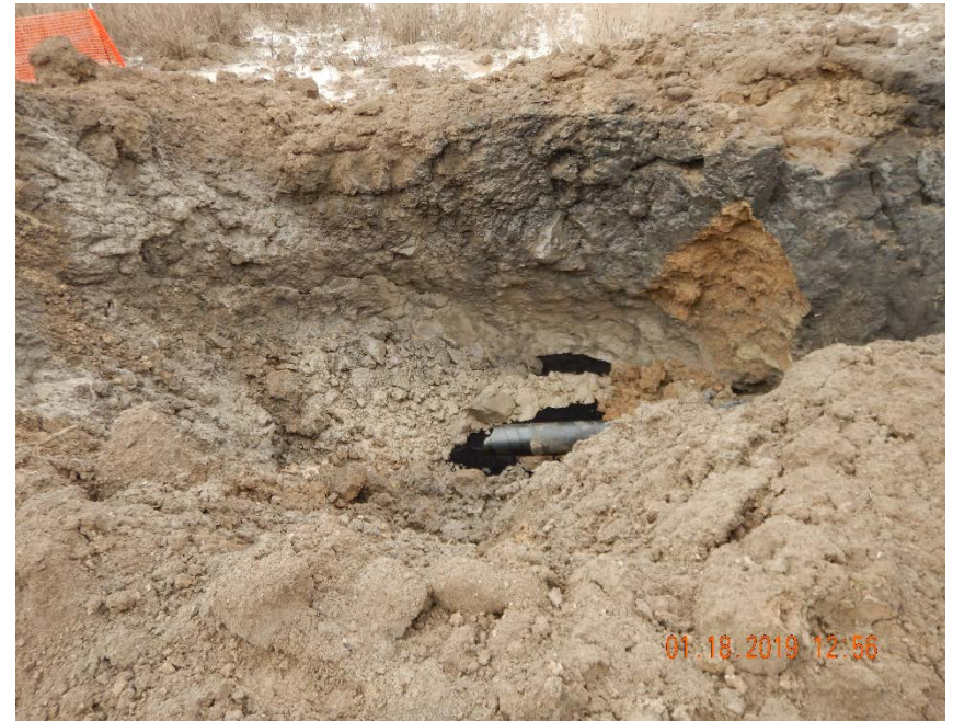
Photo #2 – View into pipeline excavation from east side. Note exposed 16" pipeline and condensate present in base of excavation.
