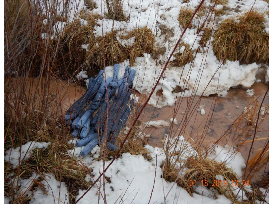
Photo #4 – Absorbent booms had been installed inside of irrigation ditch from previous photo along a fenceline located approximately 300' southeast of pipeline excavation.
