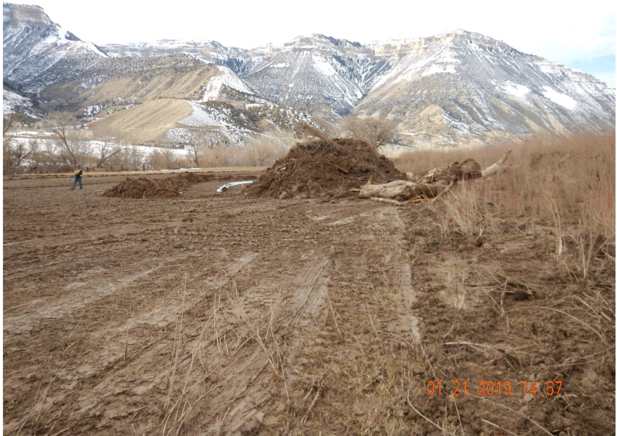
View of West Stockpile (looking north) with absorbent boom and earthen berm
