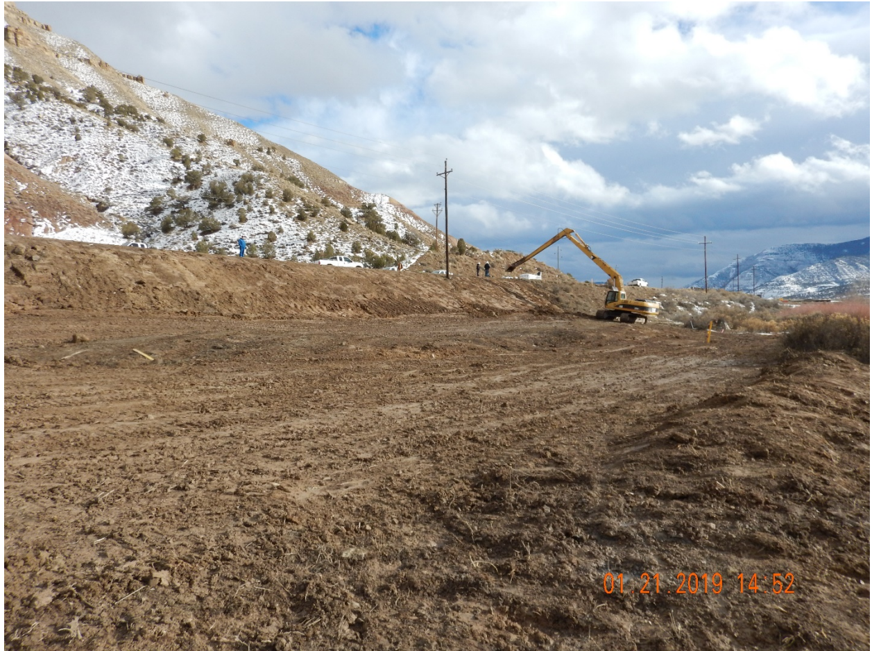
Excavator scraping surface impacts along slope leading to Co Rd 215 (looking south)
