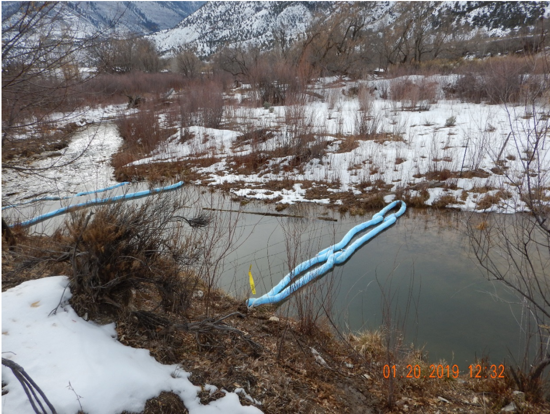
Additional booms installed downstream from confluence area
