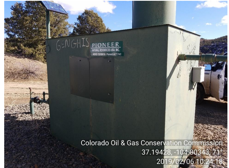
PHOTO 2: WELL SIGN/METER HOUSE/SIGN NOT POSTED OR INACCURATE INFORMATION/NO EMERGENCY CONTACT NUMBER
