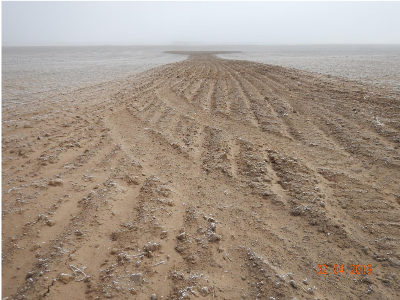
Photo 2: Photo taken from the access road, facing east. Access road appears unchanged since previous inspection; Unable to find evidence that compaction alleviation has been conducted in accordance with 1004.a on access road.
