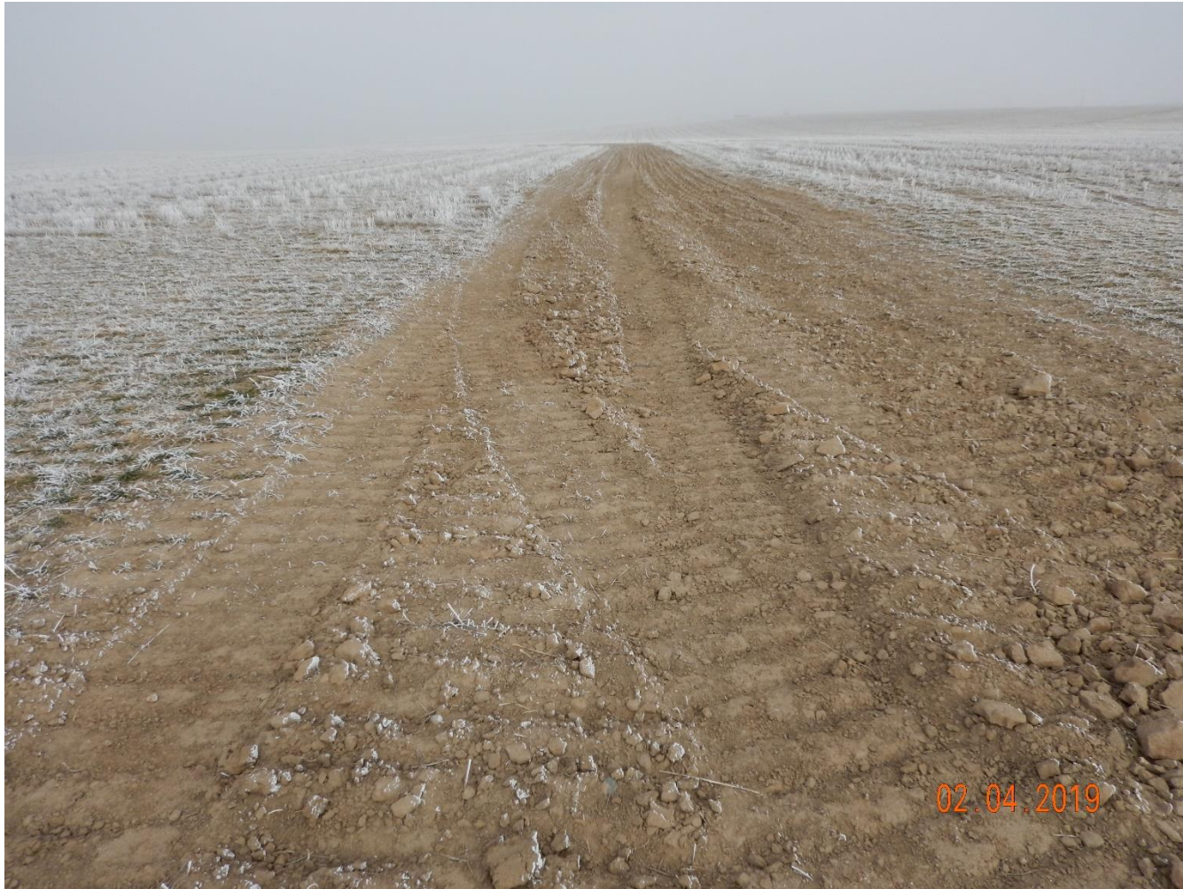
Photo 4: Photo taken from the access road, facing north. Access road appears unchanged since previous inspection; Unable to find evidence that compaction alleviation has been conducted in accordance with 1004.a on access road.
