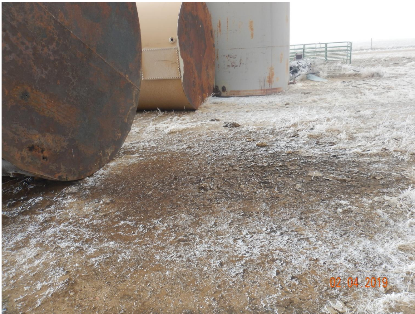
Photo 5: Photo taken from the battery location, facing. Photo shows tank laying on side. Base of tank appears to have a hole. Photo also shows contaminated soils at tank base have not been remediated/removed.
