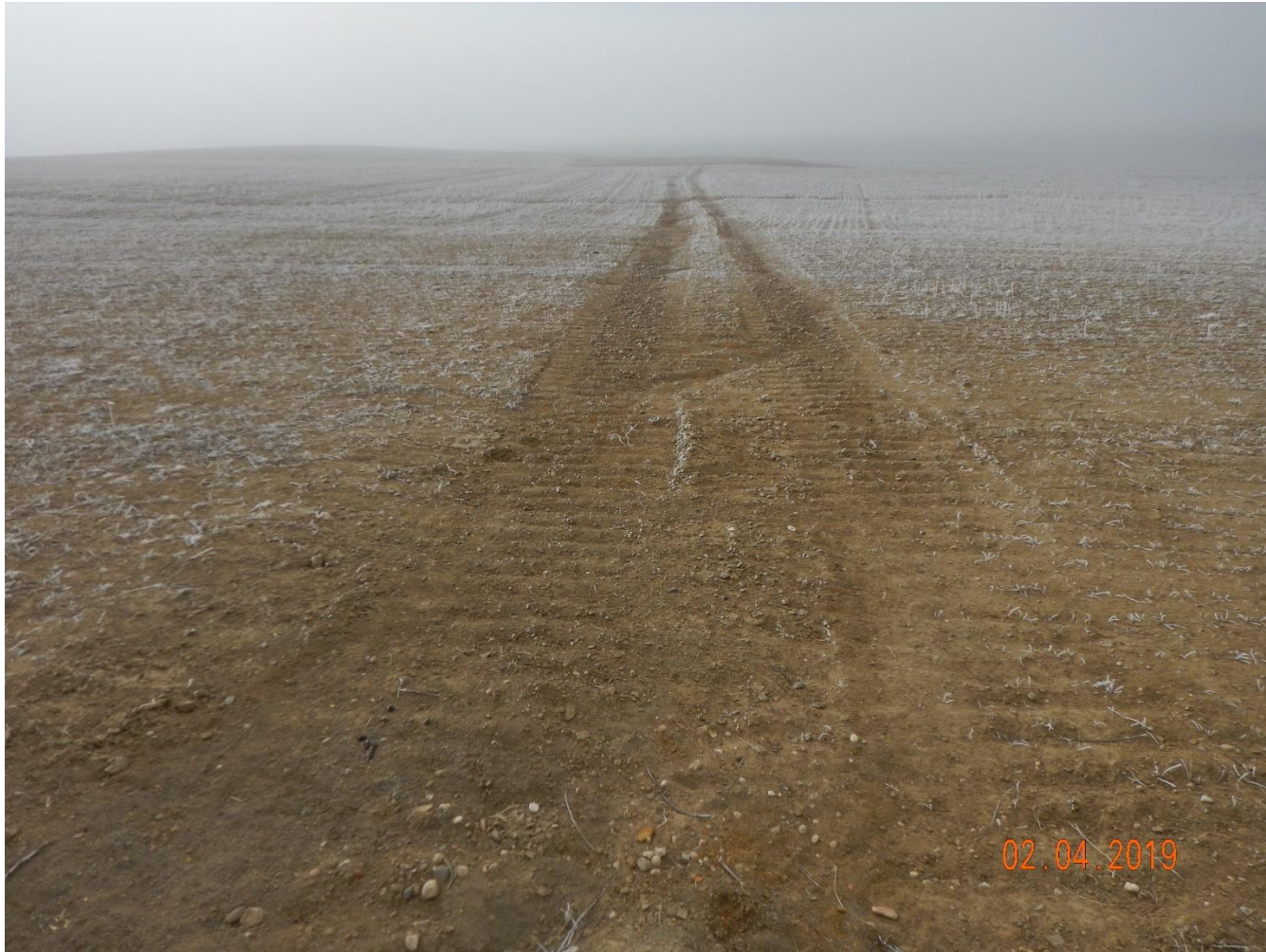
Photo 5: Photo taken from the access road, north of the location, facing south. Photo shows access road. Unable to find evidence that compaction alleviation has been conducted in accordance with 1004.a
