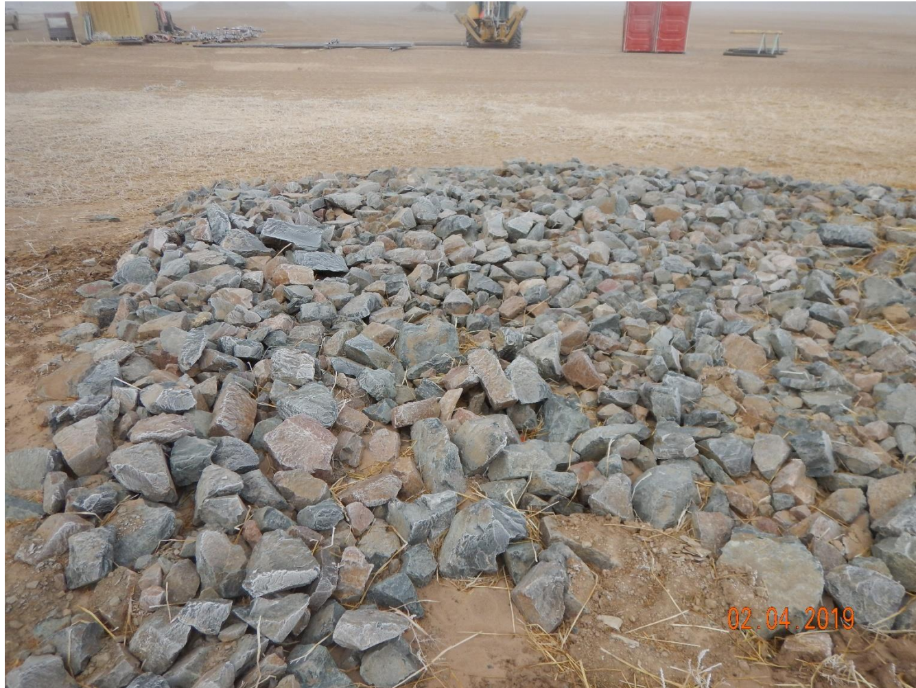
Photo 3: Photo taken from the southeast end of the location. Photo shows the outlet of the sediment pond/trap has been armored. Outlet protection appears to be sufficient and in proper functioning condition.
