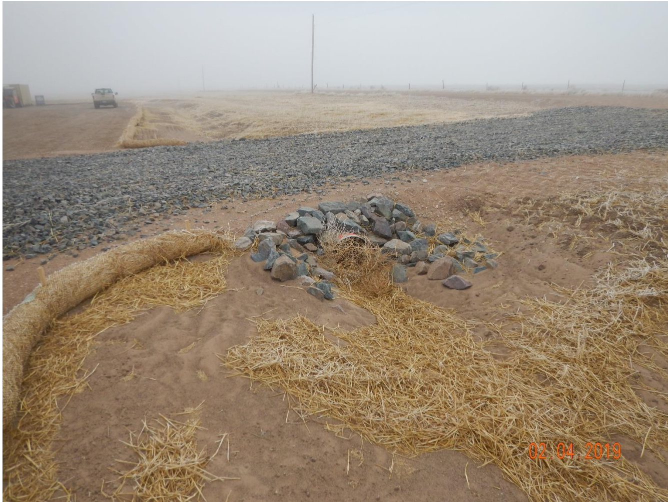
Photo 13: Photo taken from the south end of the location. Photo shows culvert and rock armoring. Photo also shows tracking pad.
