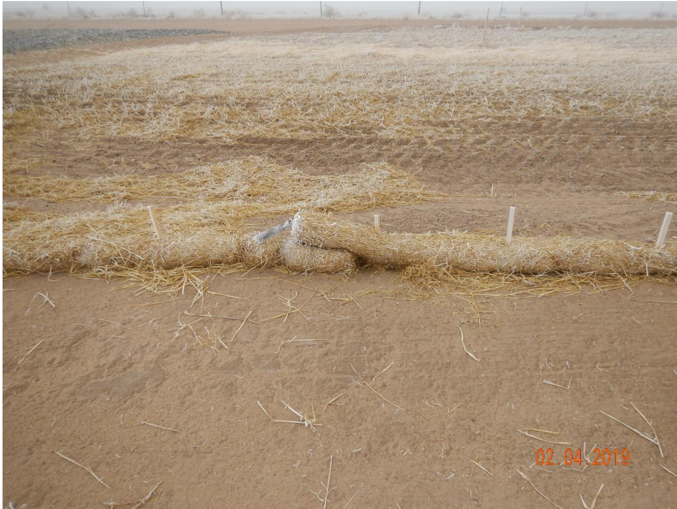
Photo 12: Photo taken from the south end of the pad. Photo shows wattles do not appear to have been installed in accordance with good engineering practice. Wattles are required to be tightly “butted” at the ends.
