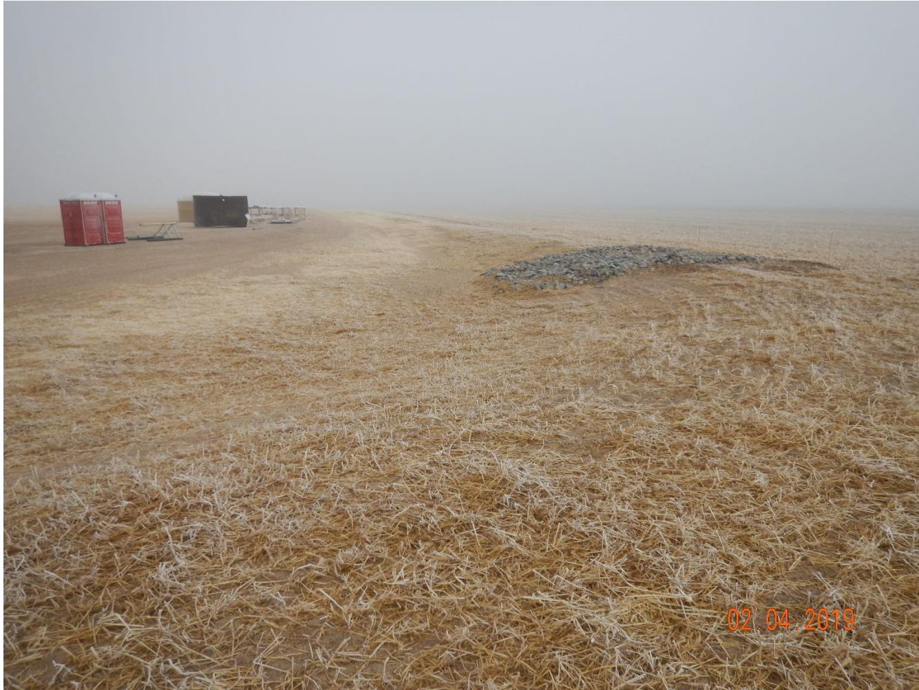
Photo 2: Photo taken from the southeast corner of the location, facing west. Photo shows perimeter stormwater ditch, and sediment pond/trap. Photo also show disturbed areas along perimeter of location appear to have been seeded and mulched.
