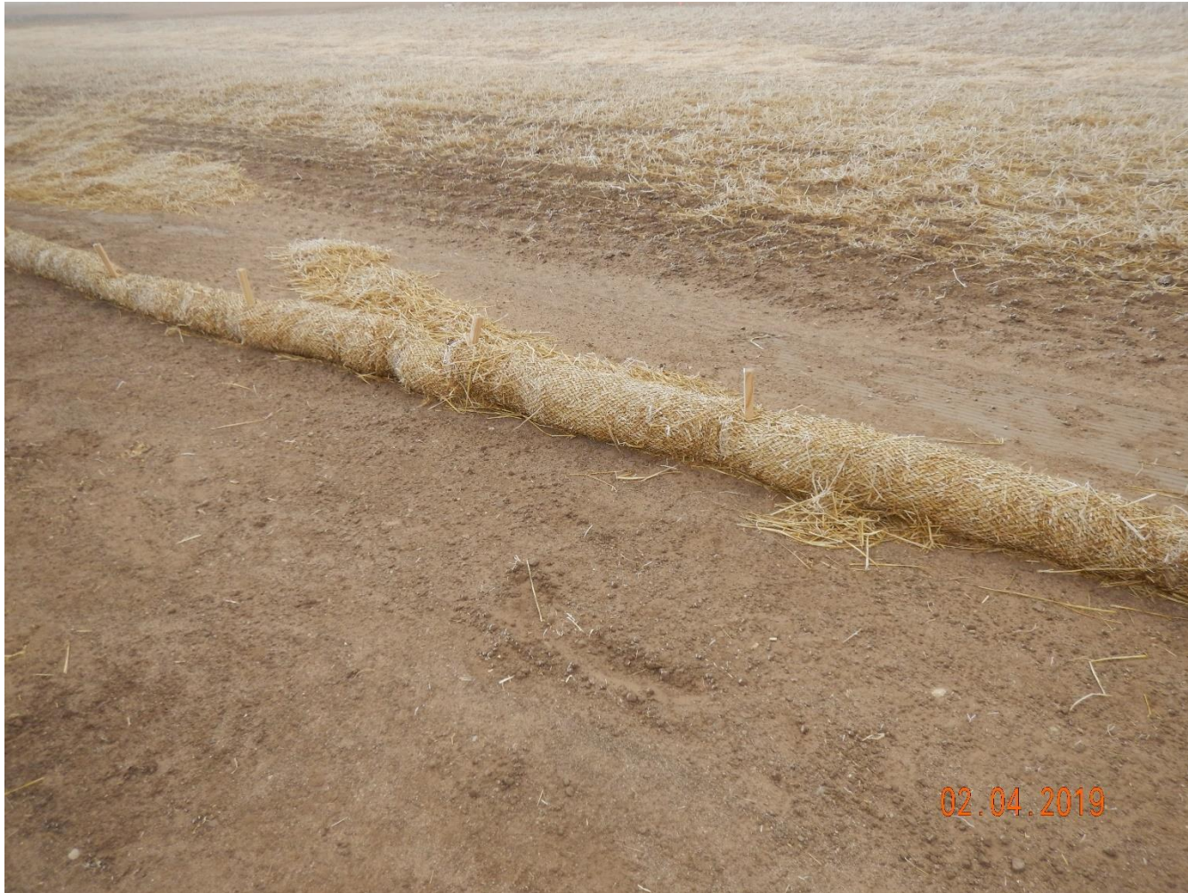
Photo 11: Photo taken from the south end of the pad. Photo shows wattles do not appear to have been installed in accordance with good engineering practice. Wattles are required to be trenched in order to be in proper functioning condition.
