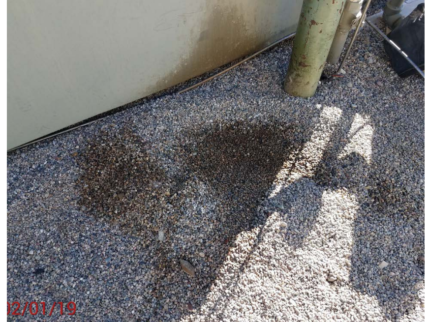
Location Photo #4, Stained material near scrubber pot not cleaned.
