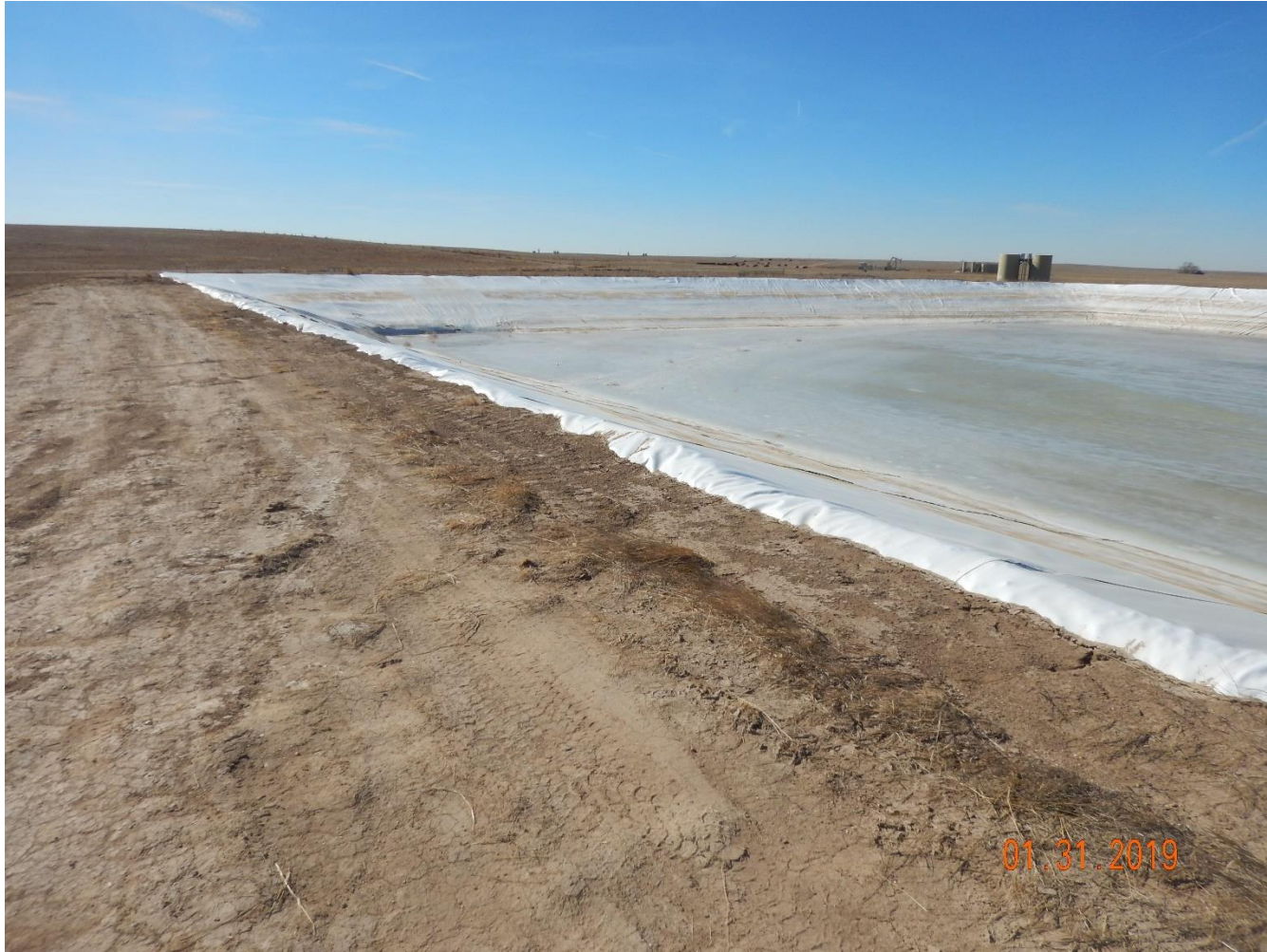
Photo 2: Photo taken from the southeast end of pit #431409, facing west. Location received an approved 502.b variance to delay interim reclamation of the location for three (3) years until 12/31/2018. Photos 2- 4 shows pit has not been closed/reclaimed.
