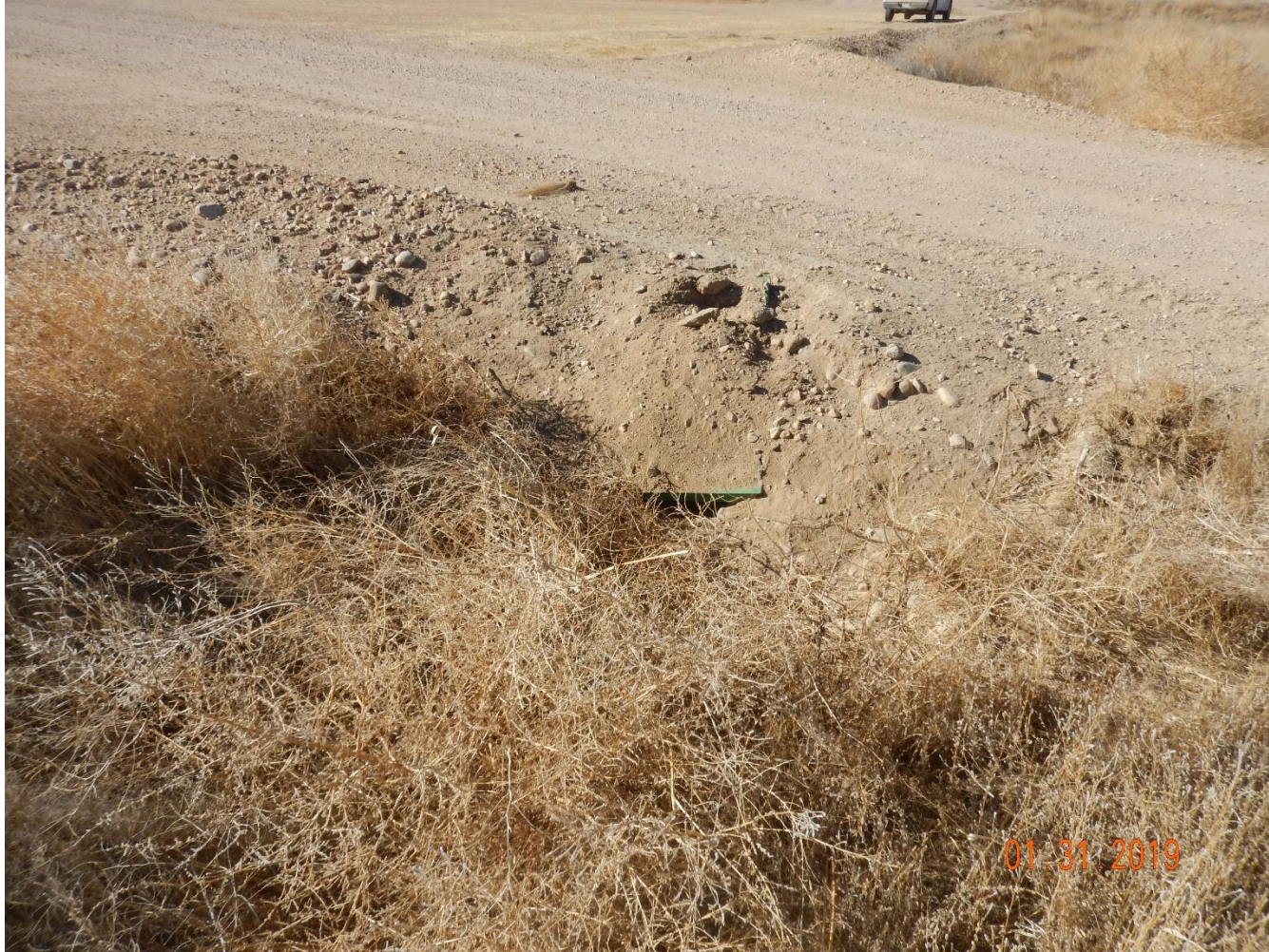
Photo 10: Photo taken from the access road on the east end of the location. Photo shows culvert has filled with sediment and no longer in proper functioning condition.
