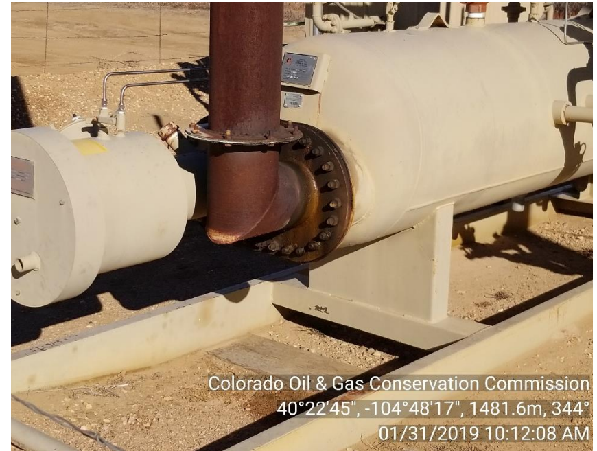
Photo 4: Appears to be stained soil from mechanical condition on east separator.
