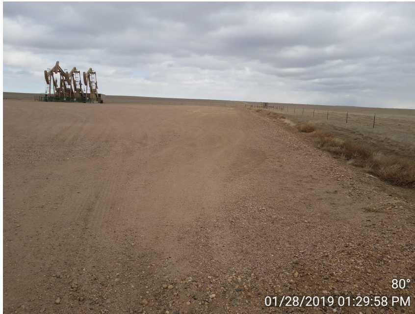
Photo 1. Photo taken from the entrance of the location, facing East. Photo illustrates the southern well pad. Operator has failed to perform interim reclamation.
