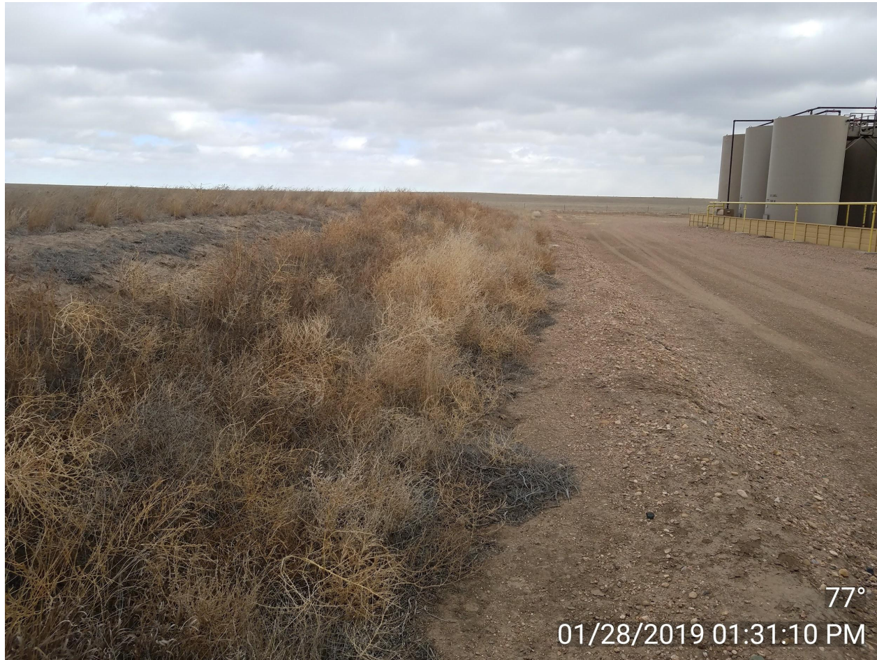
Photo 3. Photo taken from the northwestern well pad, facing East. Photo illustrates unmanaged weeds along the southern fill slope of the topsoil stockpile. Operator shall control weeds and weed debris per Rule 603.f. and comply with Rule 1002.c.
