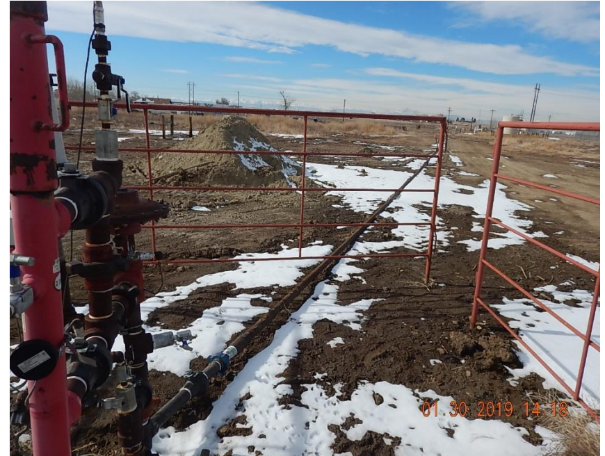
Flowline on ground surface running NW to battery
