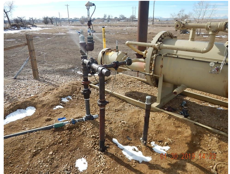
Flowline tie in at horizontal separator; also unused and unmarked flowline riser (incomplete abandonment); Riser is absent of lockout/ tagout.
