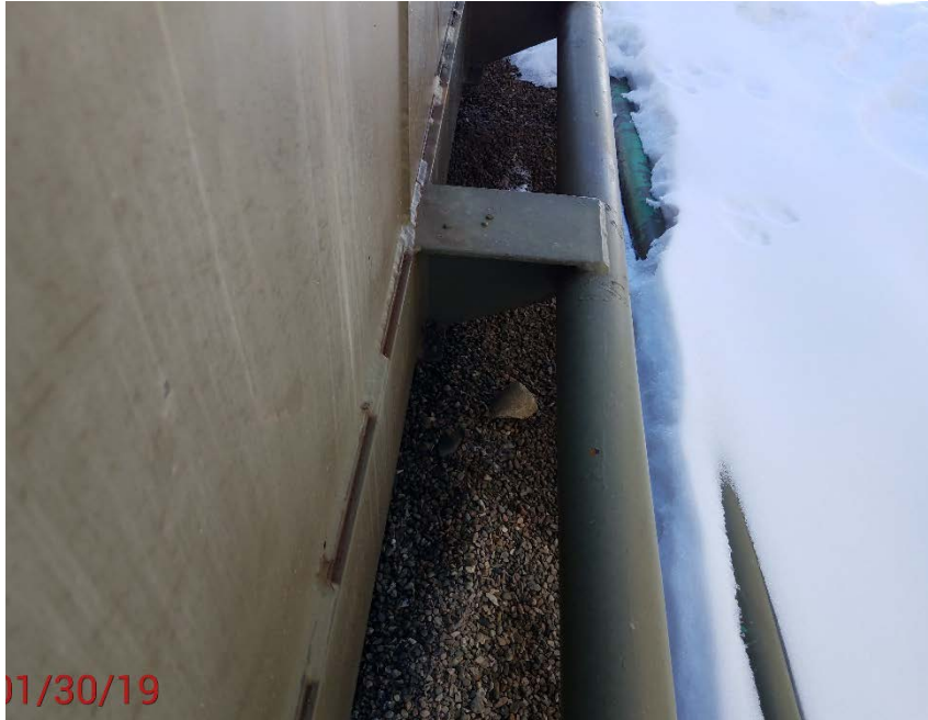
Location Photo #7, Stained rock on North end of Vertical Separators.
