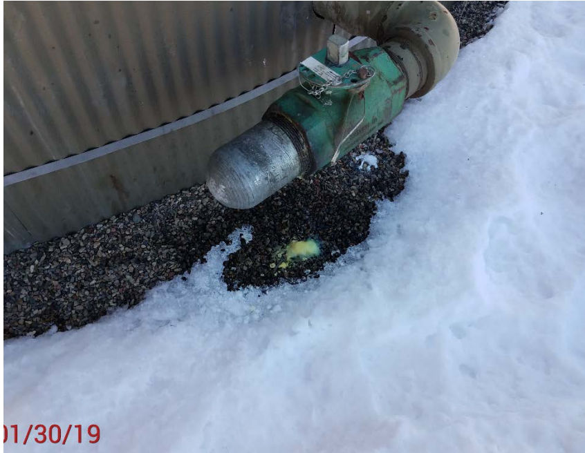
Location Photo #9, Mechanical condition of tank valve. Stained rock below valve.
