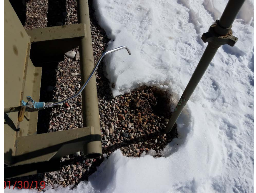
Location Photo #6, Stained rock at blowdown line from separator.
