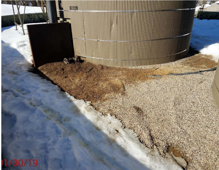
Location Photo #5, Stained material in battery containment.
