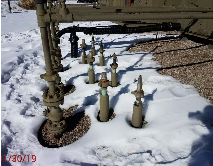
Location Photo #5, unmarked flowline risers.
