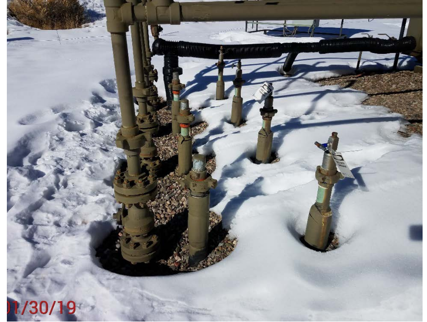
Location Photo #6, unmarked flowline risers.
