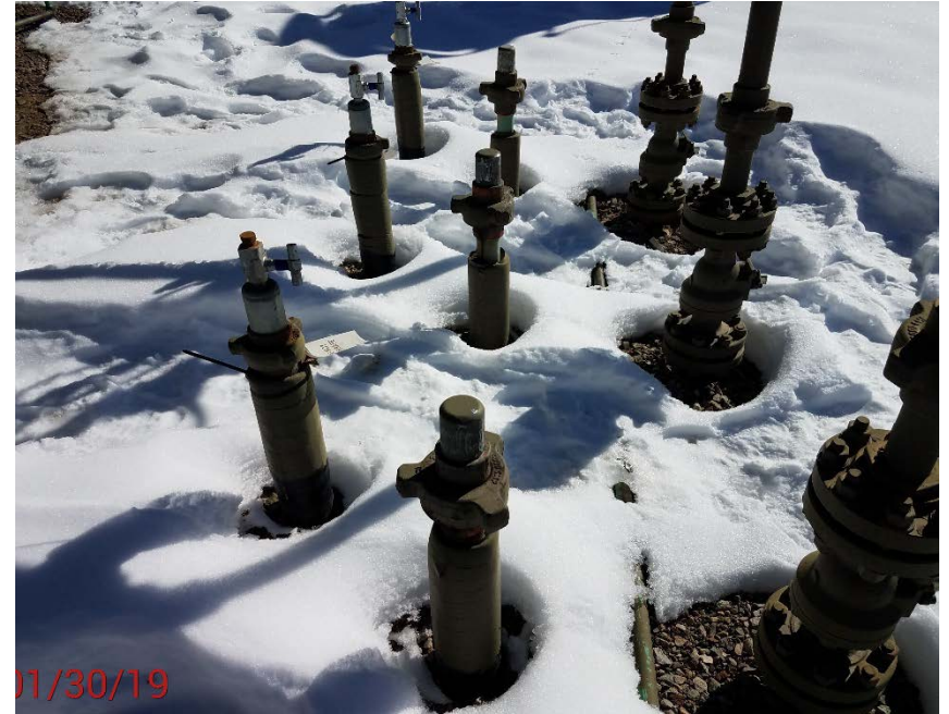
Location Photo #4, Unmarked flowline risers.
