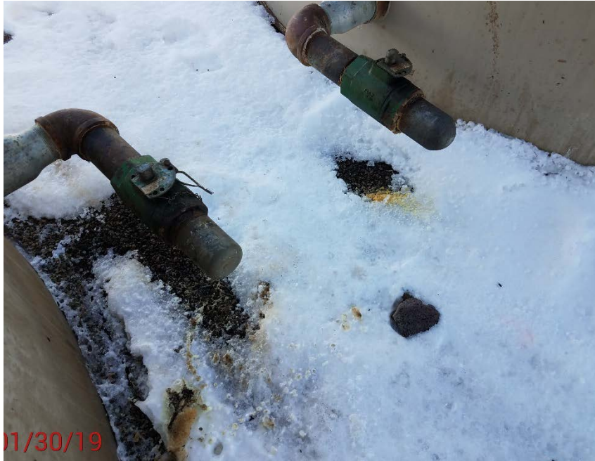
Location Photo #3, Stained soil. Mechanical integrity of valves.
