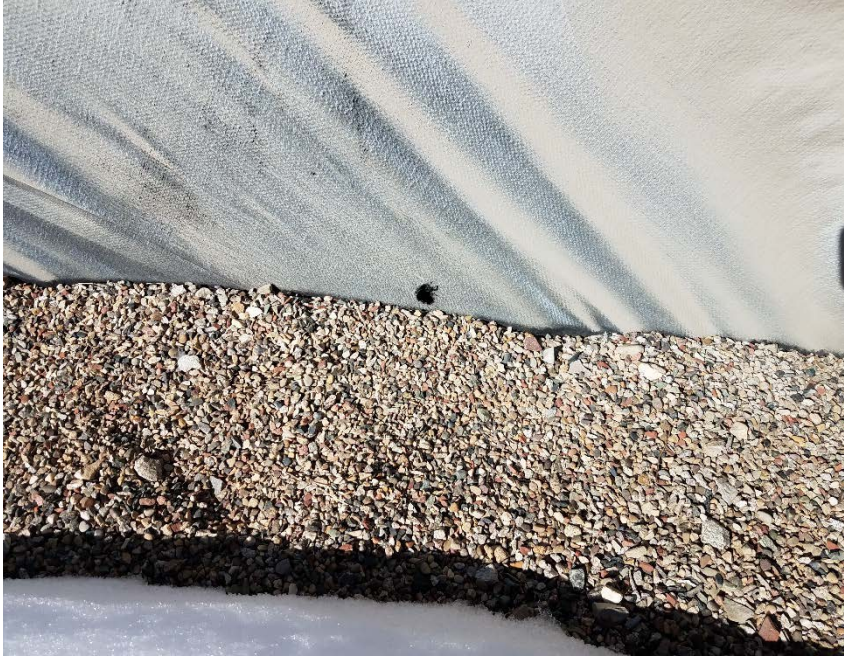
Location Photo #3, Hole in secondary containment liner.
