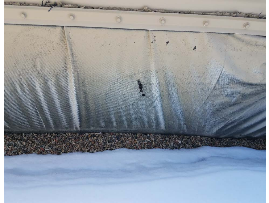
Location Photo #4, Hole in secondary containment liner.
