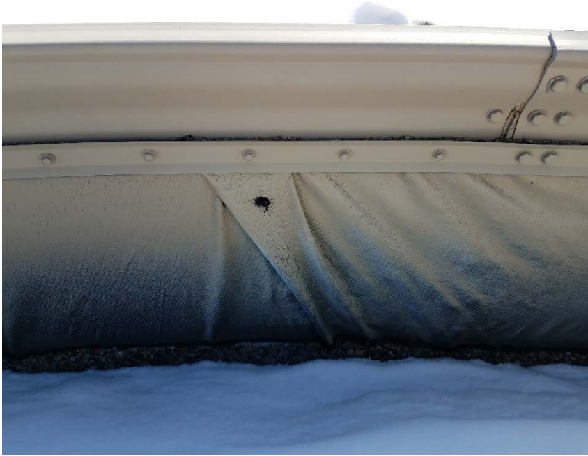
Location Photo #5, Hole in secondary containment liner.
